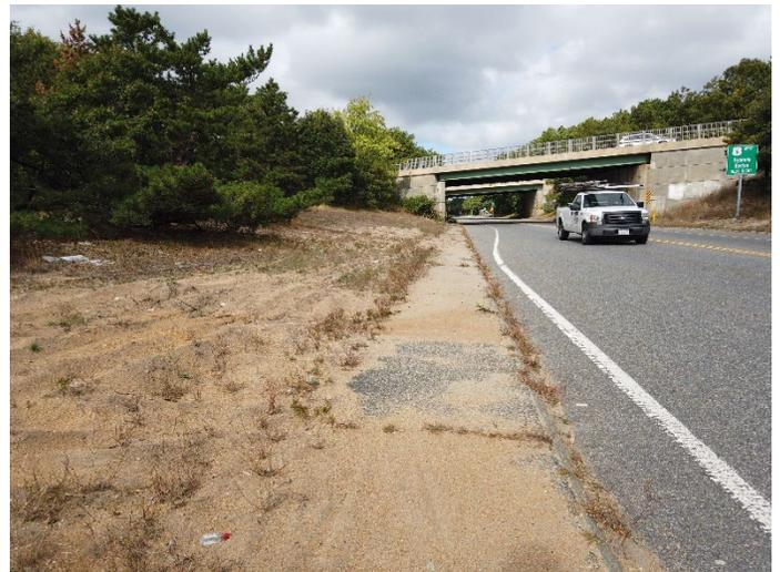
It is also recommended that MassDOT continue to clear the sand off sidewalks near the Route 6 ramps caused from runoff during rain events.
