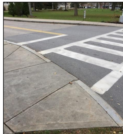
Image 3: Curb ramp along Main Street with non-compliant transition slopes.
