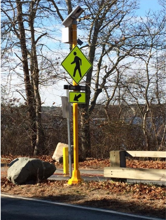
Motion activated flashing light at Harwich CCRT crossing on Rt 124
