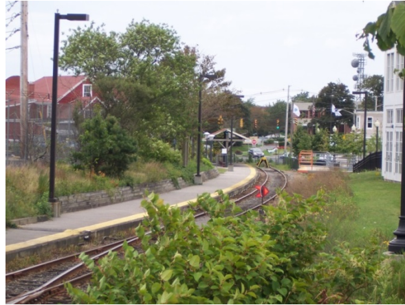
FIGURE 41. Rail Platform at the Hyannis Transportation Center
