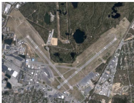
FIGURE 45. Barnstable Municipal Airport
