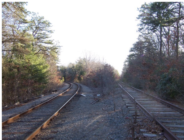
FIGURE 43. Rail Tracks at the Otis Junction
