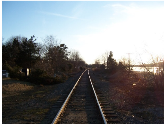
FIGURE 38. Rail Tracks West of the Sagamore Bridge
