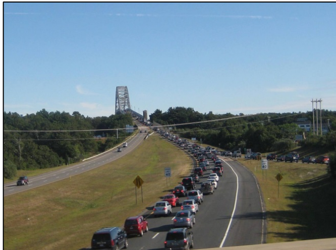
FIGURE 13. Congestion at the Bourne Bridge
