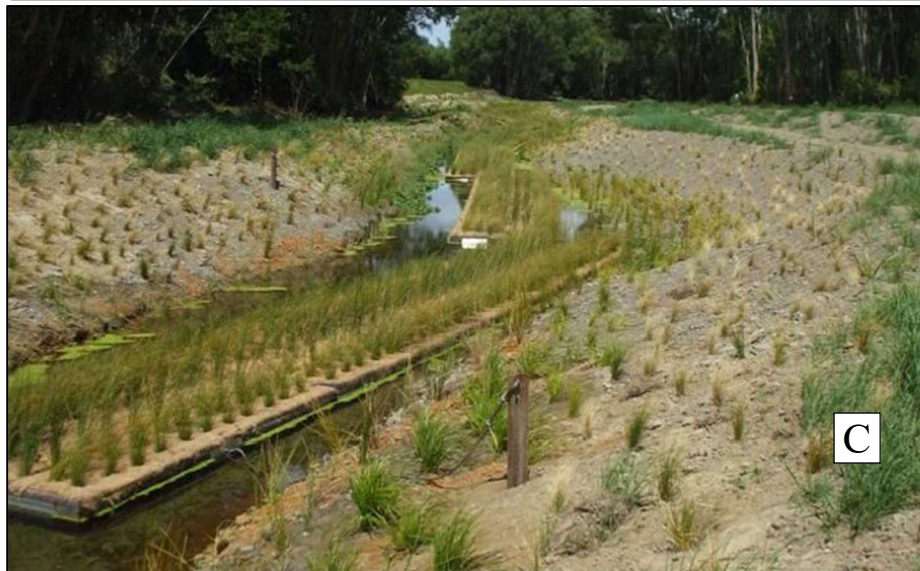
Figure V-3. Floating Wetland Examples. Floating wetlands have typically been installed in situations with high nutrient values and highly designed flows ( e.g. treating wastewater or stormwater). Current designs generally involve emergent wetland plants with roots in water growing on tethered mats or rafts (A shows typically cross-section from Tanner, et al. , 2011). Notable P removal generally require high concentrations of inorganic P, rather than the organic forms typically found in lake/ponds, and coverage of a significant portion of the water surface: B is stormwater basin in North Carolina (9% coverage pond surface by floating wetlands; Hunt, et al. , 2012), while C is agricultural drainage channel in Tukipo River, New Zealand (Tanner, et al. , 2011).
