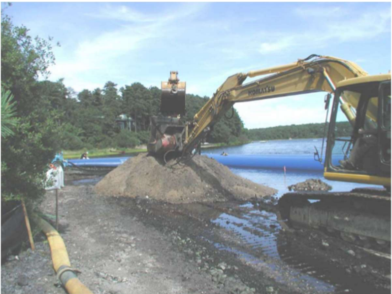
Figure V-4. Ashumet Pond Phosphorus Plume and Excavation and Dewatering to install an Iron Filings PRB to treat phosphorus. P concentrations in plume were > 5 mg/L. PRB was installed along ~300 ft of shoreline. From CH2M Hill (2005).
