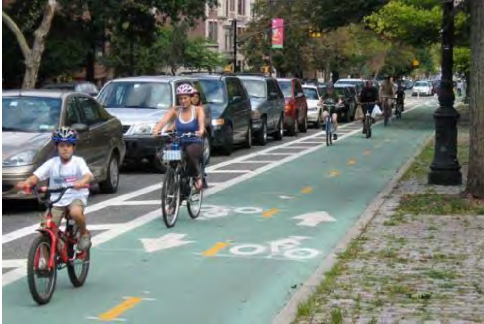
Figure 13 - Conversion of Motor Vehicle Lane to Bicycle Path in Minneapolis
