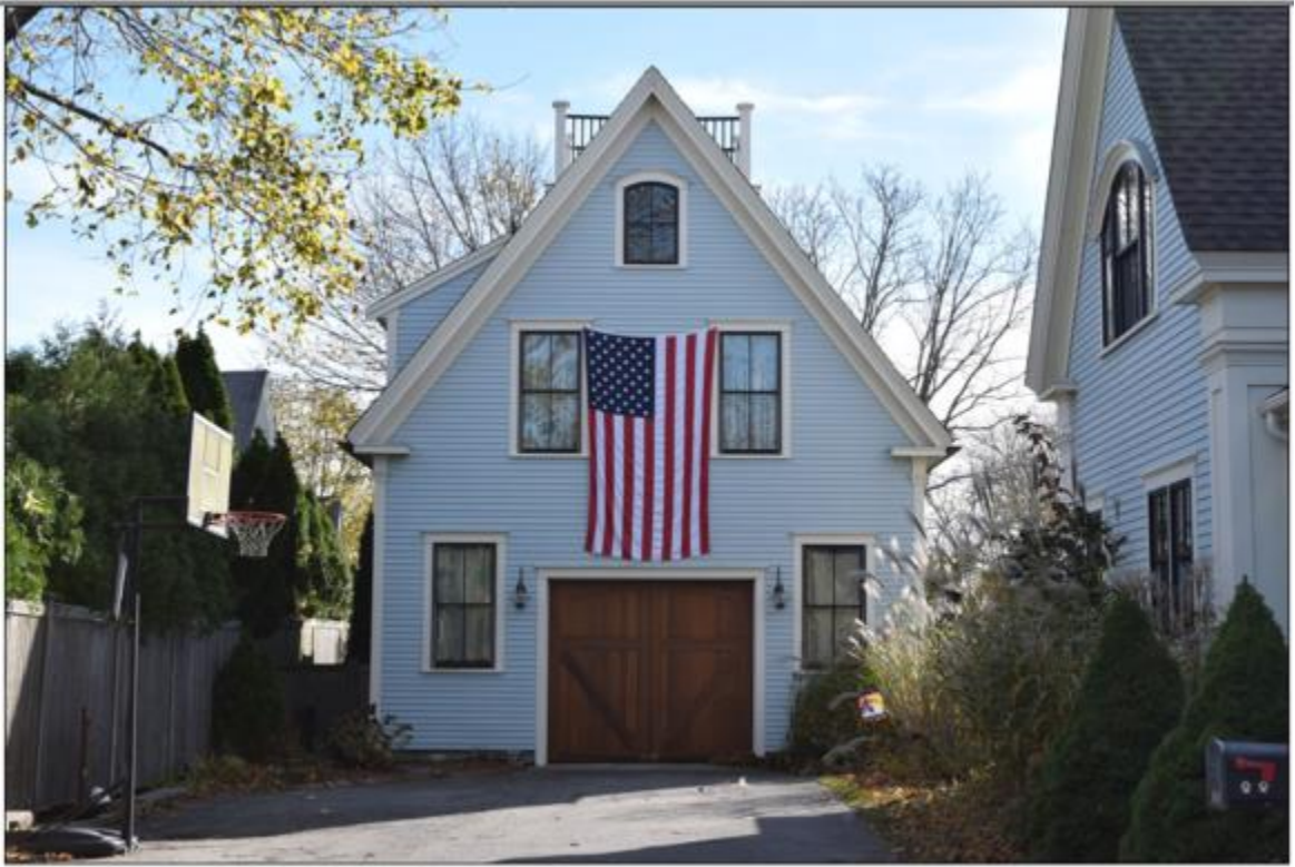
Photo 3. Barn at 275 Old Main Street, looking southwest.
