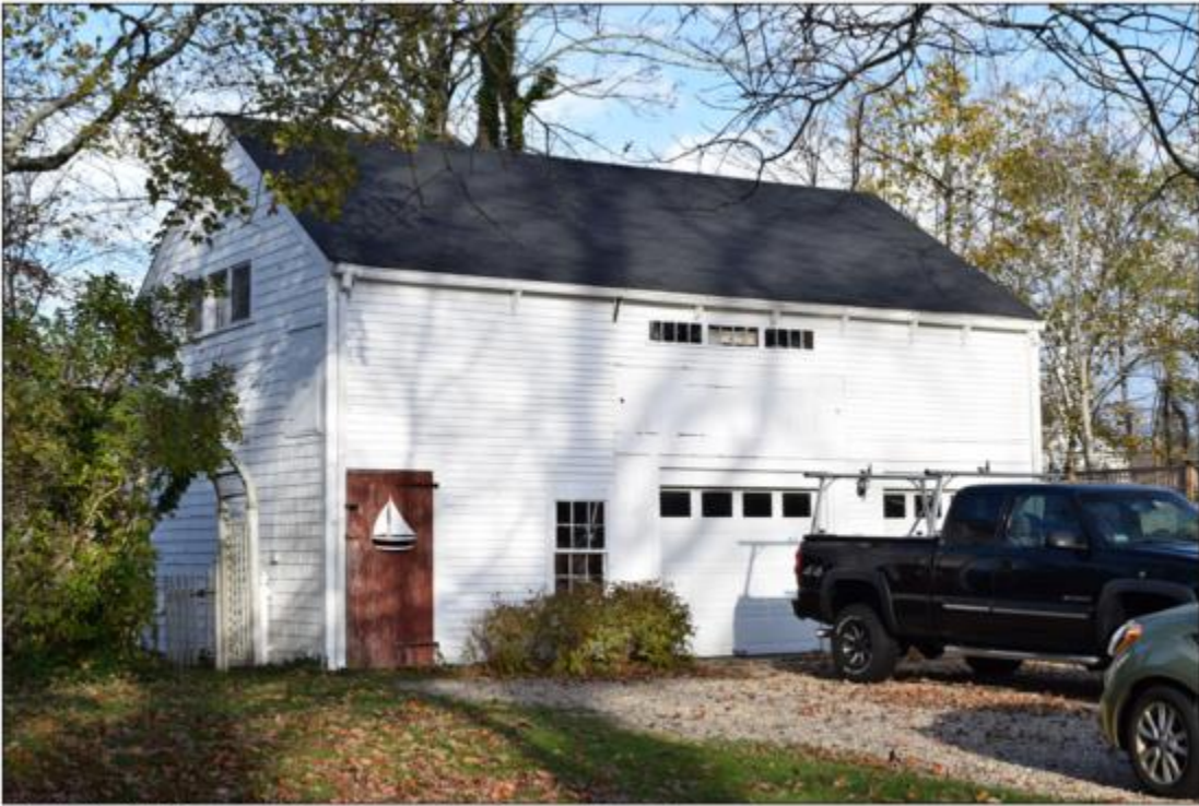
Photo 4. 33 Pleasant Street barn, looking northwest.
