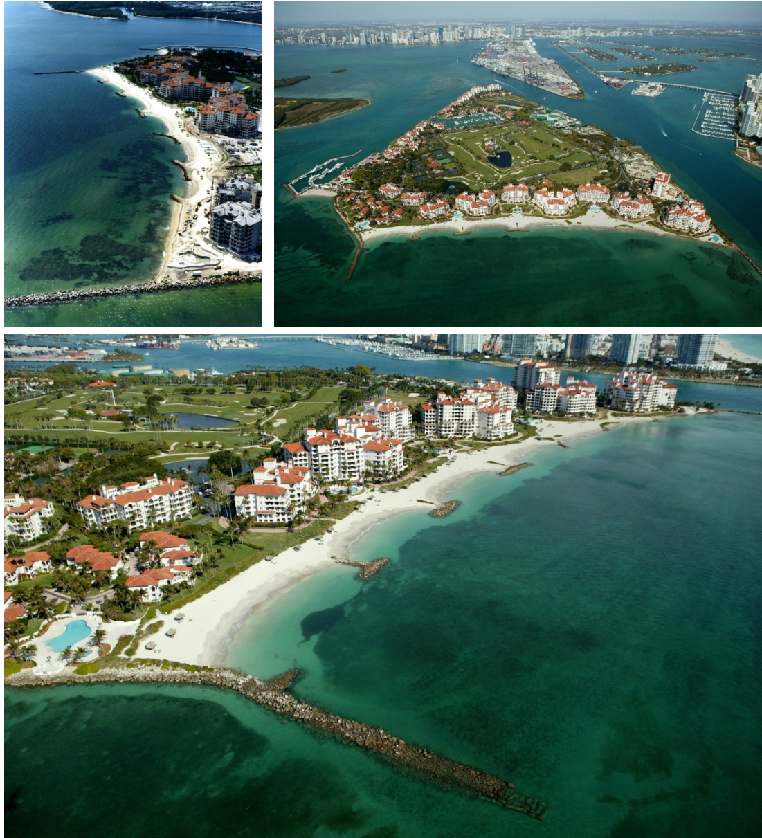
Figure 11: Fisher Island, Florida. Seven T-head and spur groin structures, with sand fill, constructed in 1991 to restore a beach eroded after the construction of Government Cut at Miami Beach in 1904.
