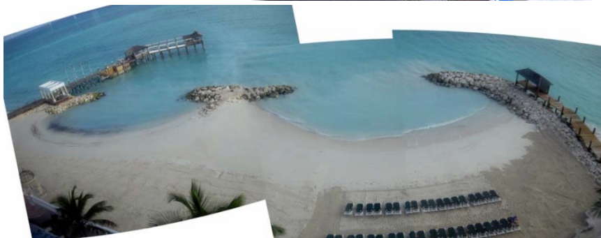
Figure 10: Sandals Royal Bahamian (Nassau, Bahamas). An existing breakwater and groin were partly removed and reconfigured to build two pocket-beach embayments with central T-head groin and sand fill in 2009, and eliminating the daily accumulation of detrital seagrass. (Top and third photograph – pre-project (2004 & 2008). Second and bottom photograph – post-project (2015 & 2010).
