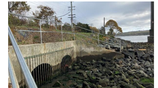
Fig. 3.6 – Existing drainage outfall and riprap
