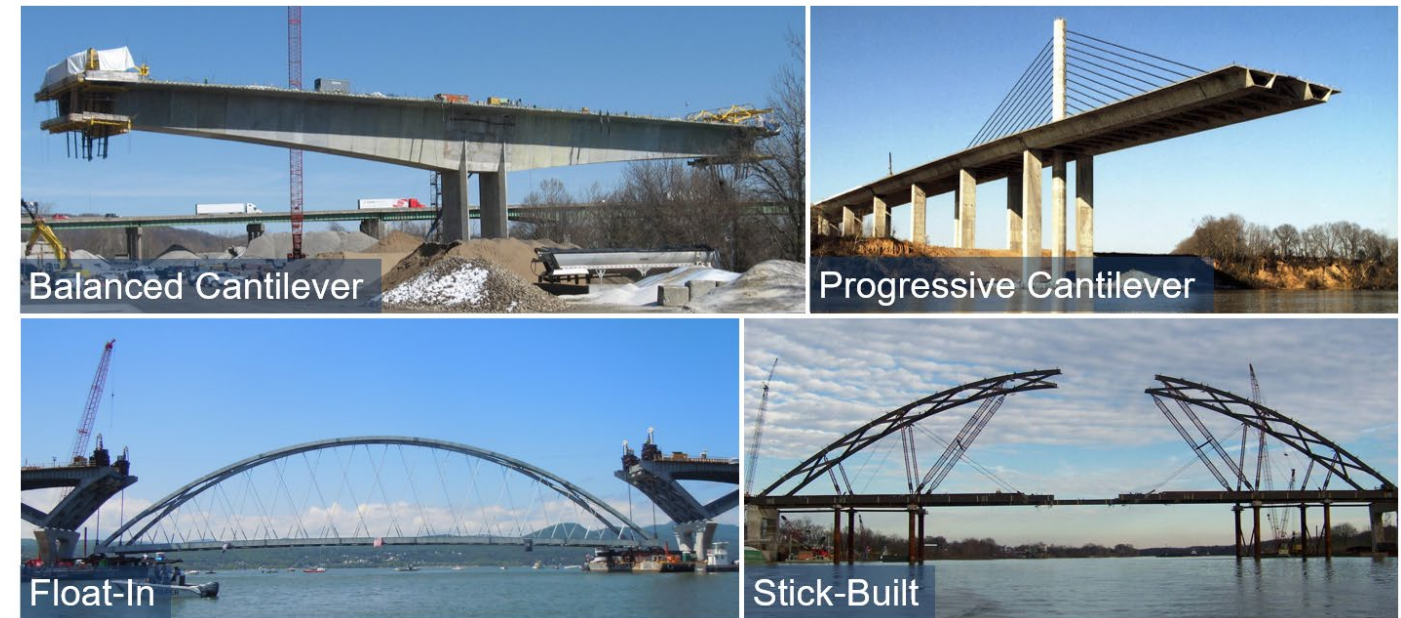
Fig. 3.5 – Main Span Superstructure Construction Methods
