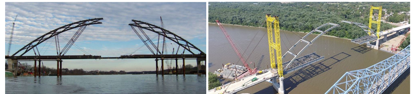
a) Temporary Piers
