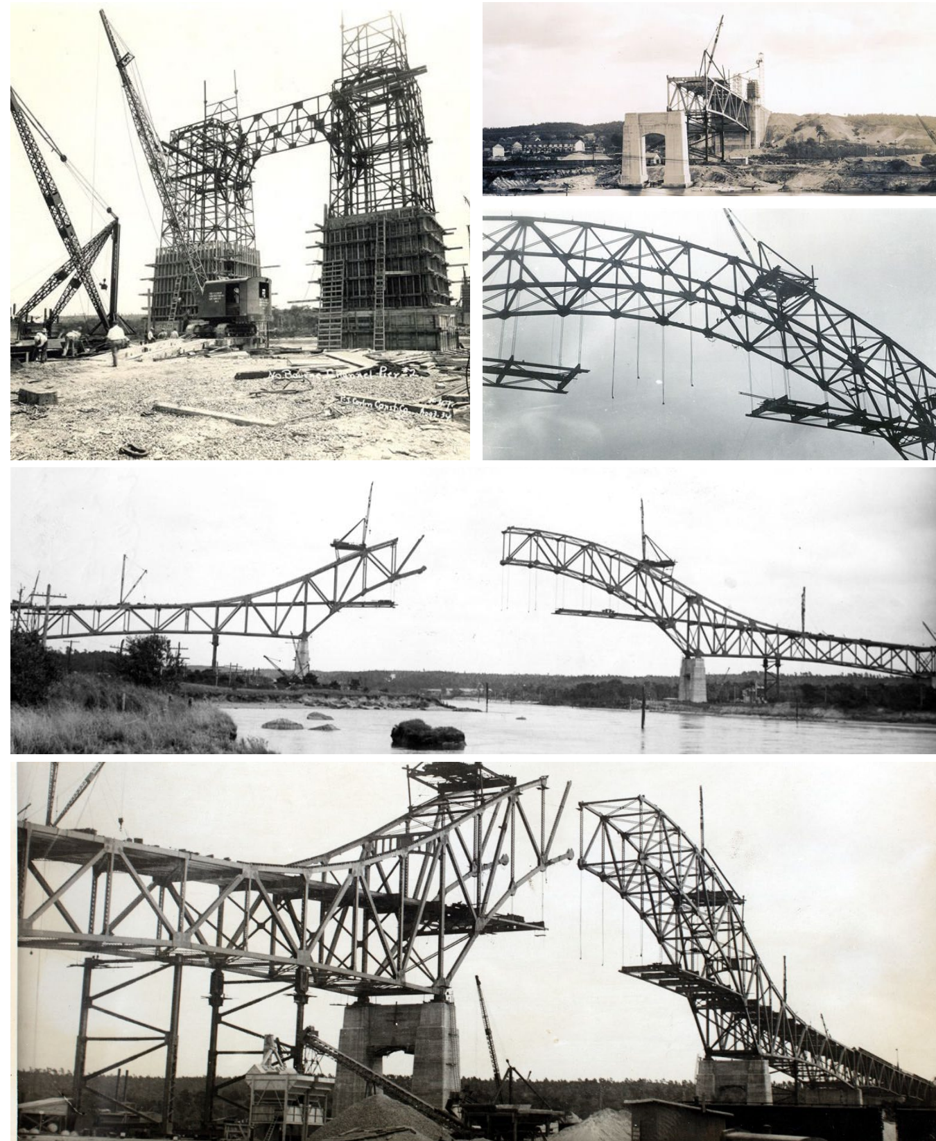
Fig. 7.3 – Historic photos showing erection of Bourne and Sagamore Bridges (c. 1934)
