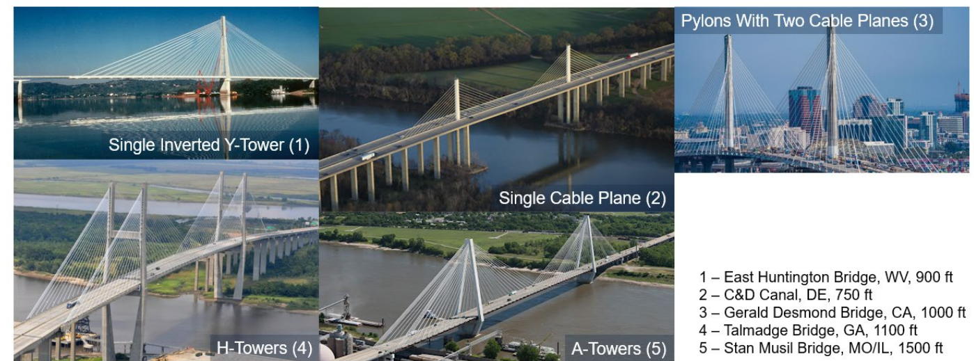
Fig. 2.12 – Representative Examples for Cable-Stayed Bridge Options
