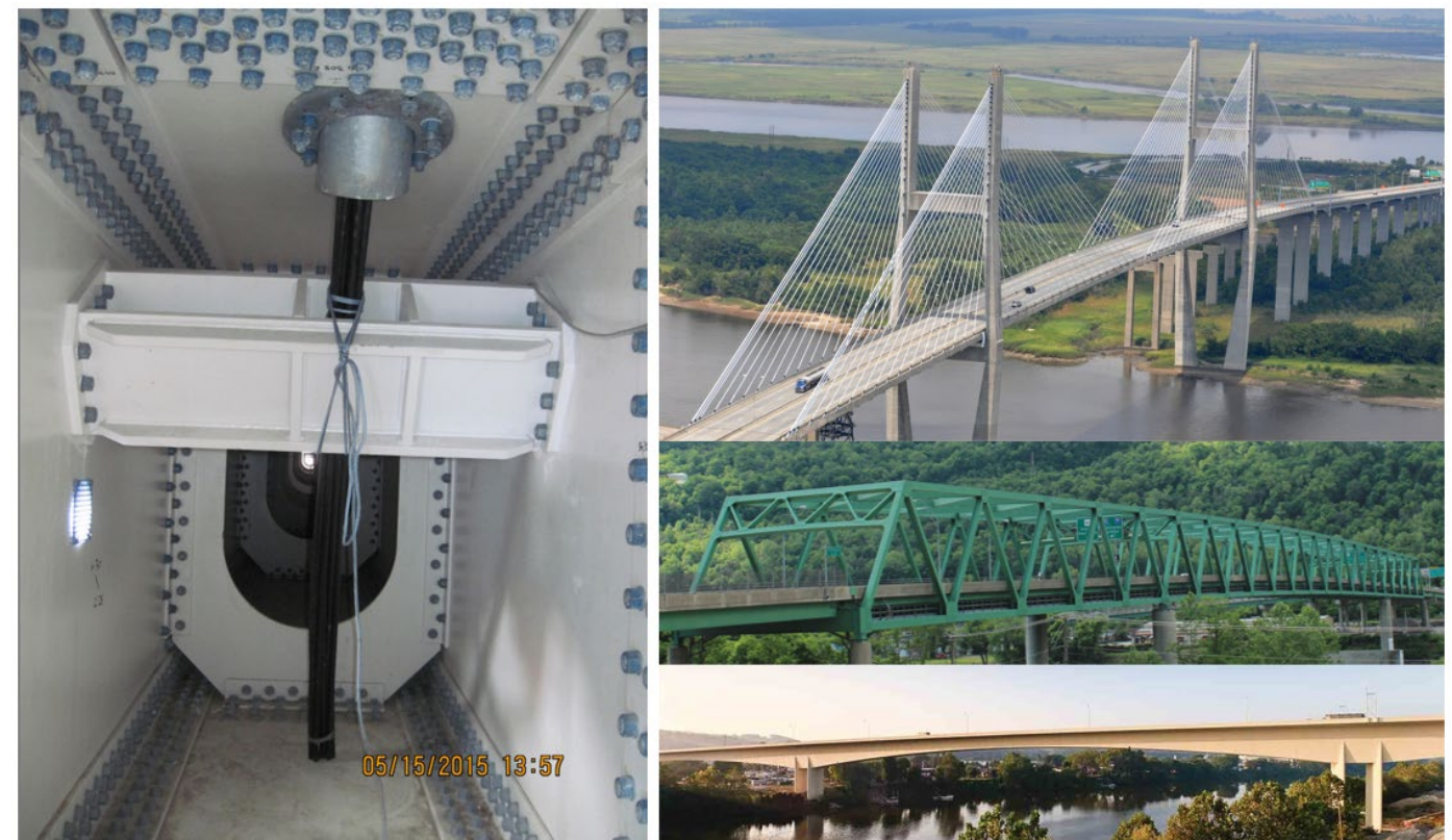
Fig. 3.8 – Inspection and Maintenance
