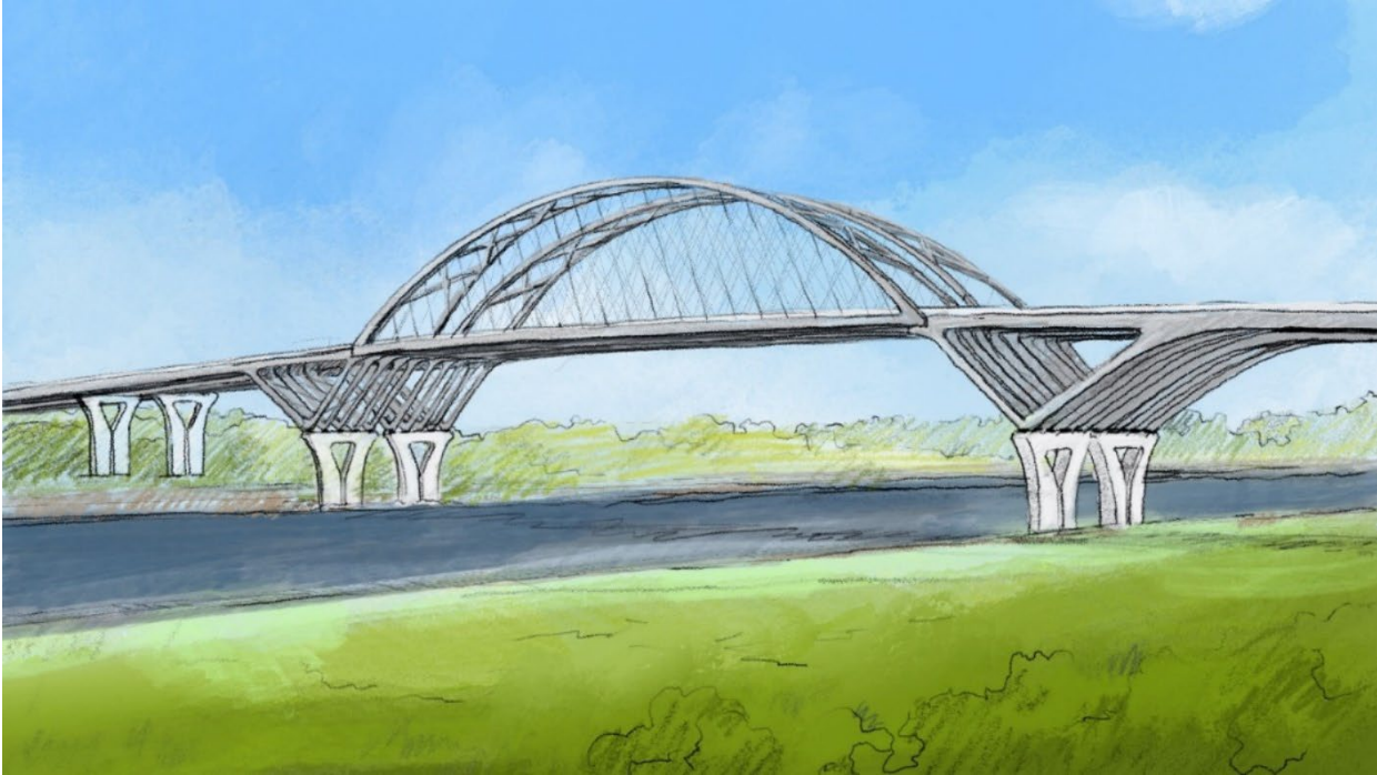
Figure 2-1. Conceptual Rendering of the Tied-Arch Bridges Preferred Alternative – Cape Cod Canal Viewpoint
