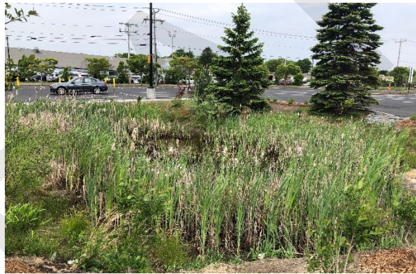
Figure 31. Bioswale/Rain-Garden in at the Hyannis Transportation Center
