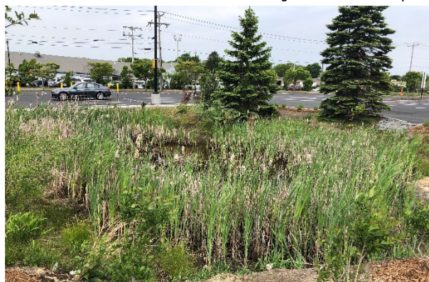
Figure 32. Bioswale/Rain-Garden in at the Hyannis Transportation Center
