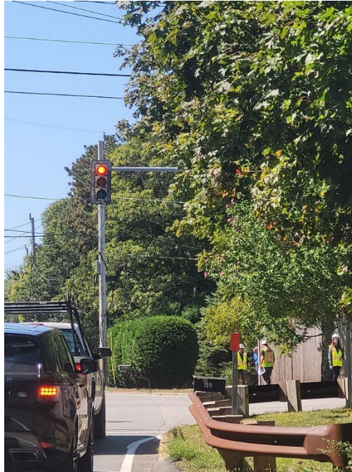
Figure 4: Drivers View of Traffic Signal Head Obstructed – Queen Anne Road Westbound
