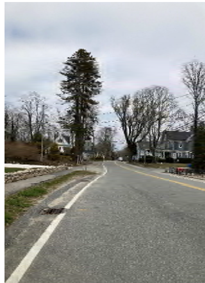
Image 13: Storm Drains on Route 28A As It Widens North of Old Dock Road
