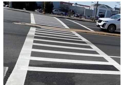
**Image 9: Crosswalk obstructed by a drain and a median at the west leg of the Cape Cod Mall Driveway/ Capetown Plaza intersection.**
