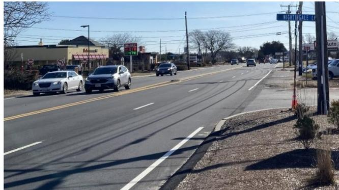
**Image 10: Intersection of Route 132 at Nightingale Lane with two lanes in each direction on Route 132 and a lack of pedestrian accommodations.**
