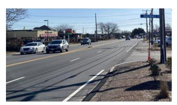
Image 10: Intersection of Route 132 at Nightingale Lane with two lanes in each direction on Route 132 and a lack of pedestrian accommodations.
