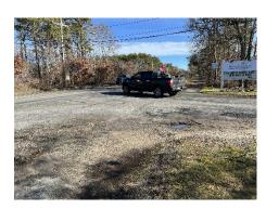
Image 6: Faded and missing pavement markings observed at the Barnstable High School access road.
