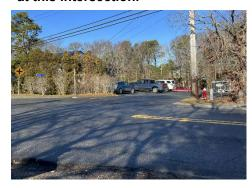
Image 22: Missing or faded fog line on Route 28, faded stop bar on Lincoln Road Extension and no visible lane markings.
