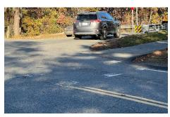
Image 21: Faded crosswalk markings and stop bar on Lincoln Road, fog lines and centerlines are also cracked at this intersection.
