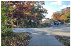
Image 19: Lack of visibility of the shared use path crossing and guardrail obstructed view.
