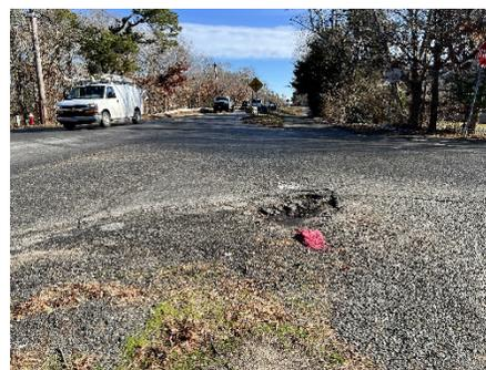
**Image 5: Lincoln Road shared use side path crosswalk, with faded pavement markings and lacking ADA compliant features**
