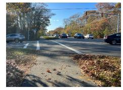
Image 16: The westbound shared use side path approach, missing the stop sign at the crosswalk and the no motor vehicles sign.
