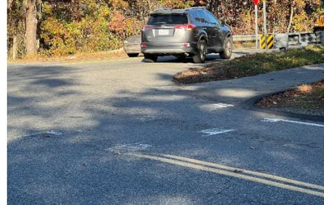
**Image 21: Faded crosswalk markings and stop bar on Lincoln Road, fog lines and centerlines are also cracked at this intersection.**
