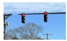
Image 9: Pitcher's Way signal heads, faded visors and no backplates.
