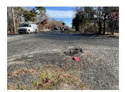
Image 5: Lincoln Road shared use side path crosswalk, with faded pavement markings and lacking ADA compliant features
