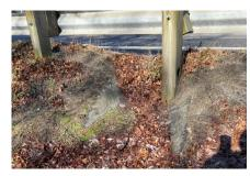
Image 7: Asphalt swale leading rainwater runoff from Route 28 onto the shared use side path.
