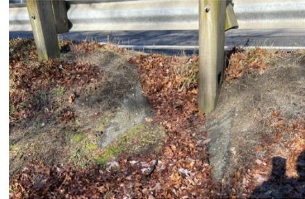
**Image 7: Asphalt swale leading rainwater runoff from Route 28 onto the shared use side path.**
