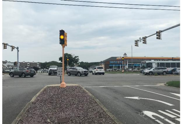
**Image 5: Pedestal Pole Mounted Signal Heads**
