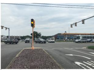
Image 5: Pedestal Pole Mounted Signal Heads
