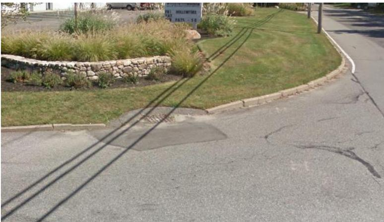
**Figure 18– Drainage on northeast corner leads to puddling during large storm events**
