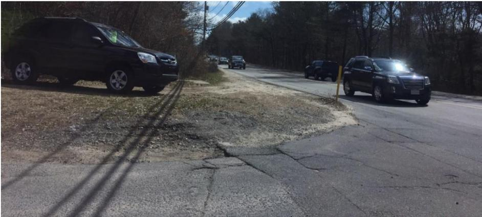
**Figure 13 – Northeast corner of intersection with poor pavement conditions and parked car blocking sight distance**
