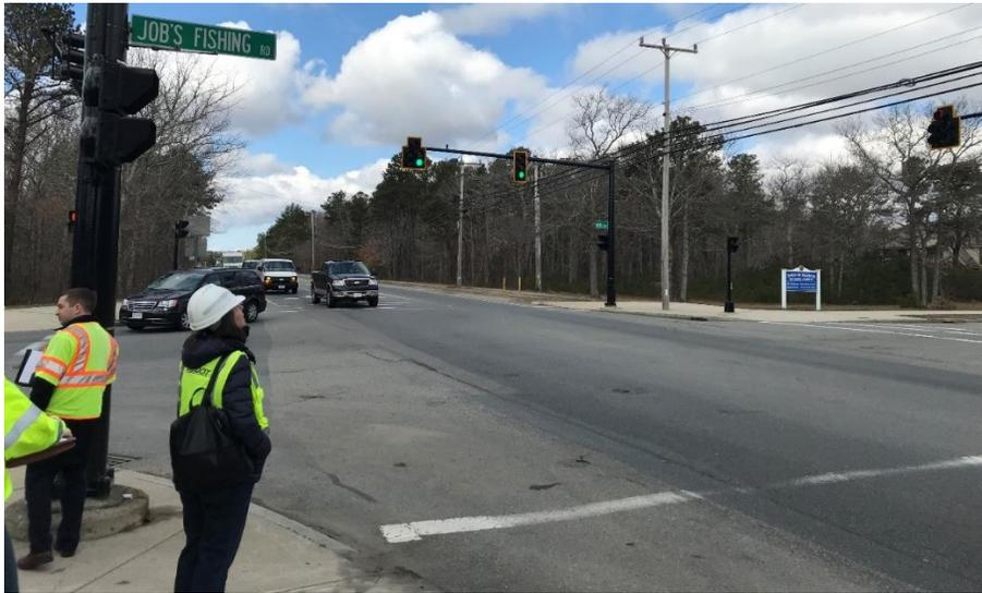
**Figure 6– Faded crosswalk markings across Route 151**
