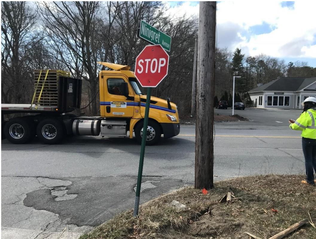
Figure 21– Undersized and bent stop sign at Ninigret Ave
