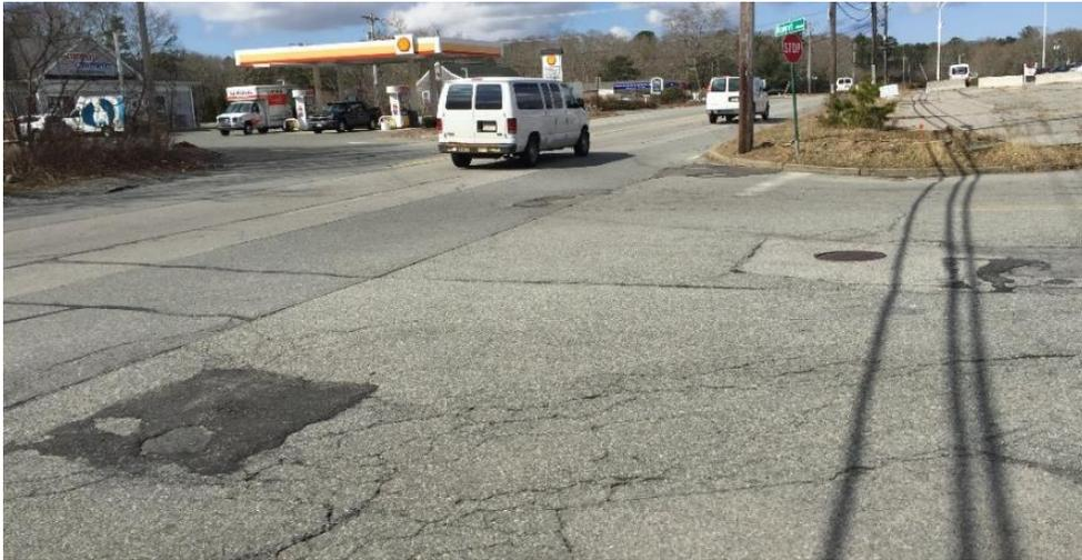
**Figure 19– Patched pavement and worn pavement marking on Ninigret Ave**
