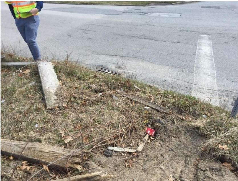
**Figure 15– Debris on northwest corner of intersection causing sight distance issues**
