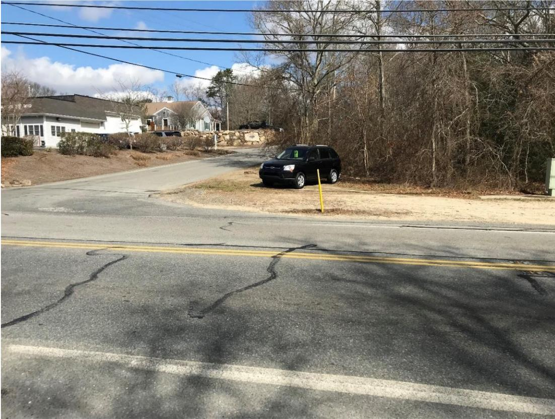
**Figure 8– Car blocking sight distance on northeast corner of intersection**
