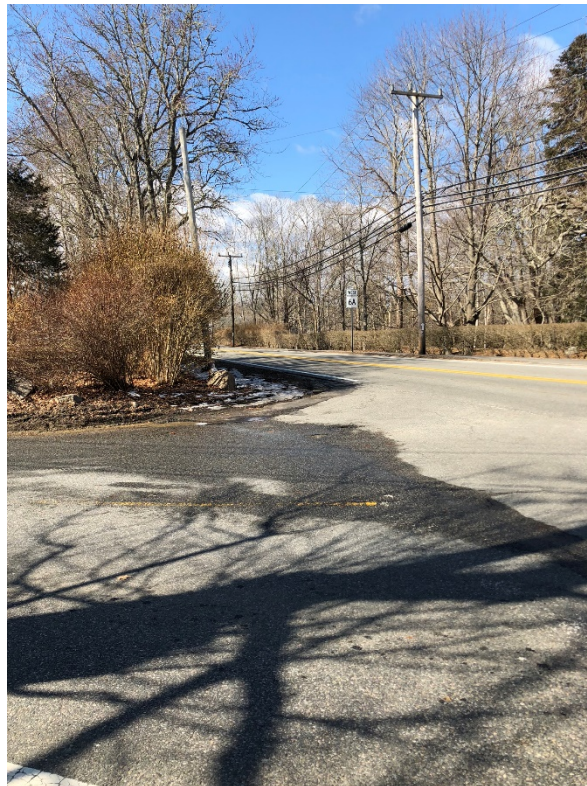
Figure 14 – Sight line obstructions in the southwest quadrant of the intersection
