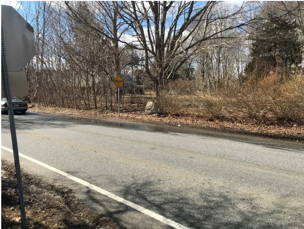
Figure 15 – Runoff flowing toward intersection on Mary Dunn Rd
