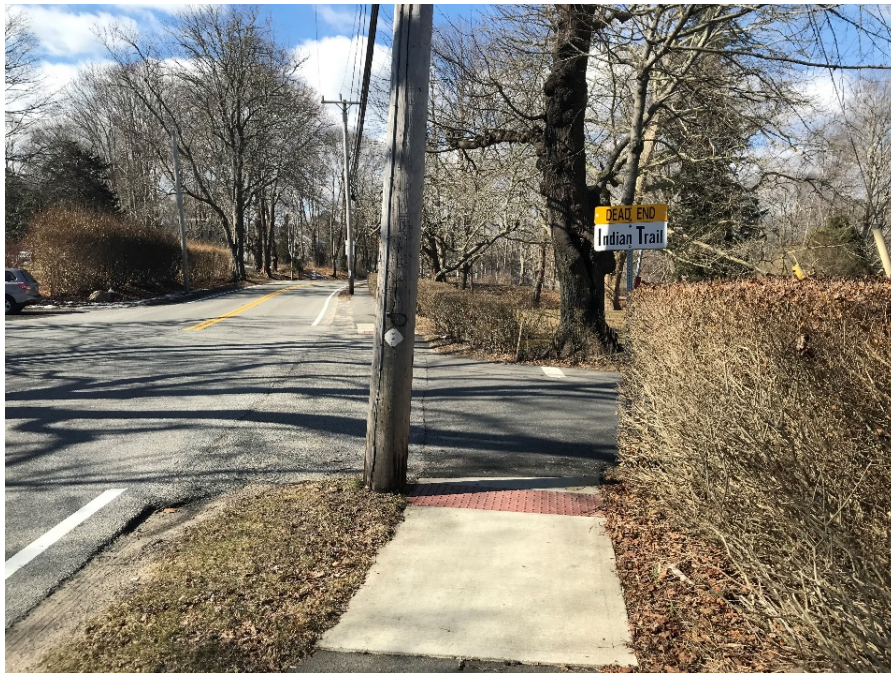
Figure 5 – Route 6A westbound approach sidewalk at Indian Trail
