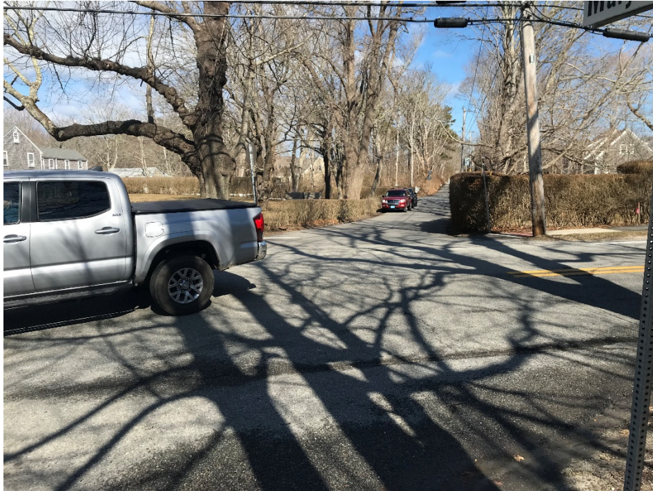
Figure 6 – Narrow road width on Indian Trail
