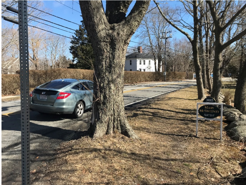
Figure 13 – Trees causing sight obstructions in southeast quadrant of intersection
