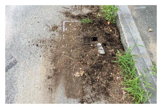
Figure 15 - Catch basin blocked by debris
