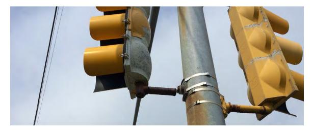
Figure 9 - Lower signal connecter arm rusted through and separated from pole on signal head in the northeast quadrant
