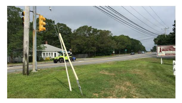
Figure 14 – Potential sight obstructions in northeast quadrant of Nauset Road intersection - utility pole and guy wires
