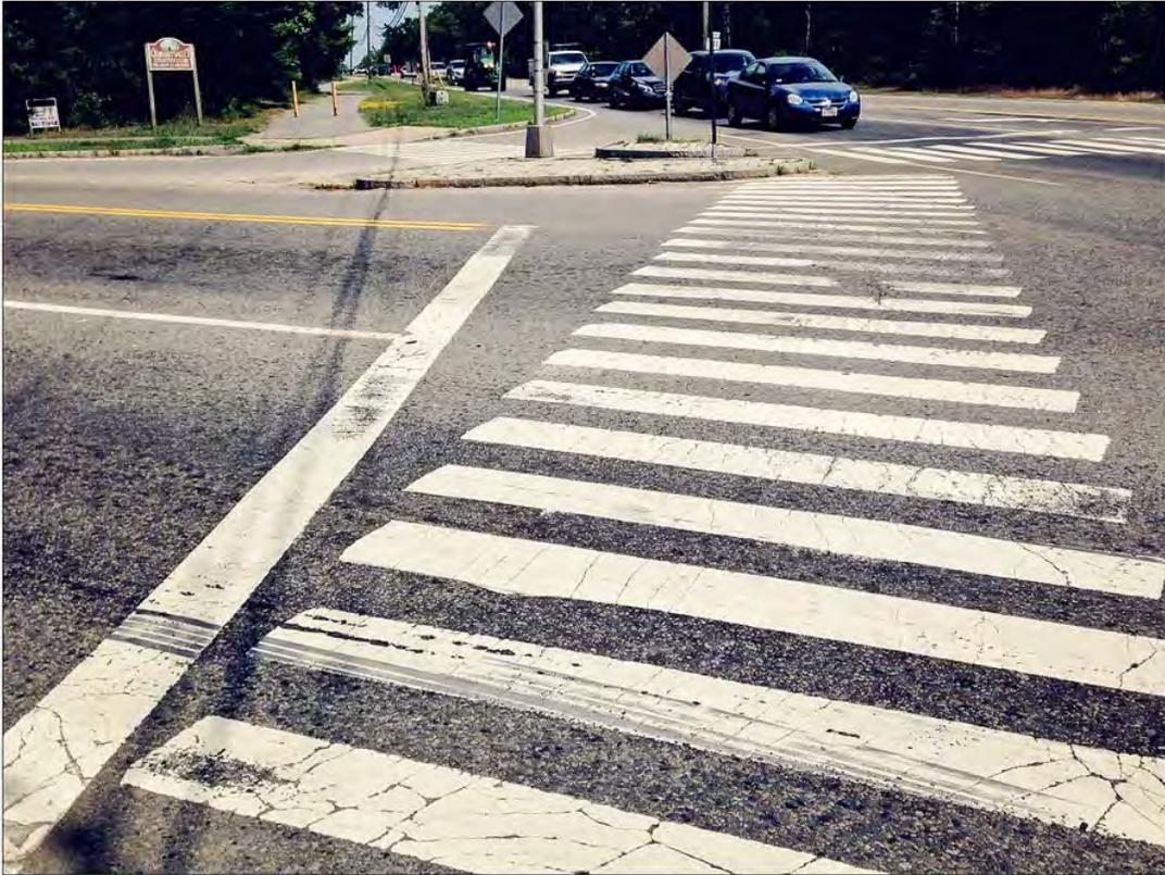
Pedestrian accommodation crossing Old Barnstable Road going east along Route 151 without handicap accessibility on the pedestrian island and directing pedestrian into incoming vehicular traffic heading west along Route 151.
