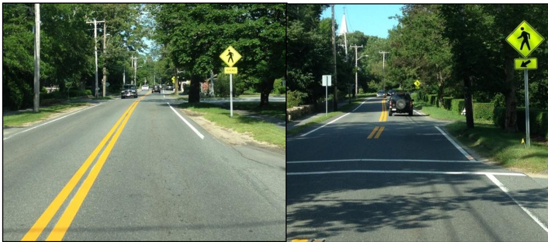
FIGURE 2. STRIPING AND PEDESTRIAN SIGNAGE IMPROVEMENTS
