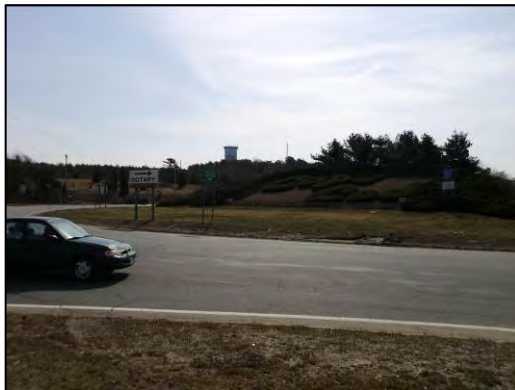
The vegetation in the center of the Bourne Rotary may be distracting, and may restrict sight lines of entering traffic.
