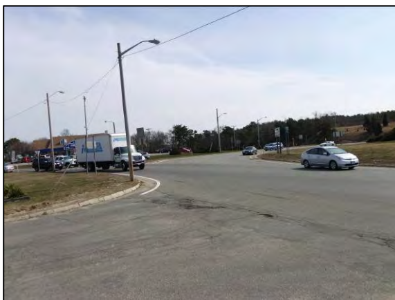
There are no longitudinal lane markings or arrow markings within the Bourne Rotary to guide vehicles through the rotary.
