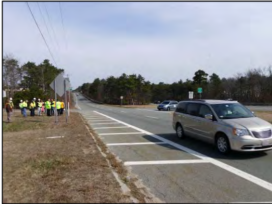
Sight lines to the north of the turnaround in the vicinity of Waterhouse Road are obstructed by vegetation in the median and a crest vertical curve.
