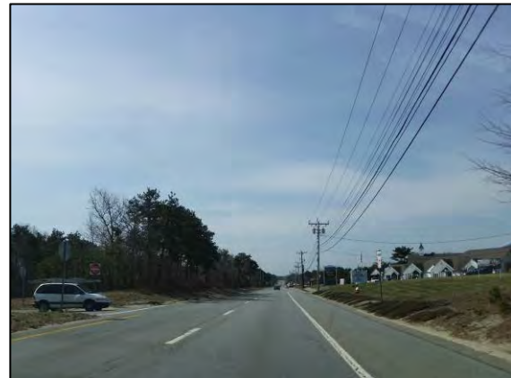
Most turnarounds between the northbound and southbound directions on Route 28 do not provide an acceleration lane.
