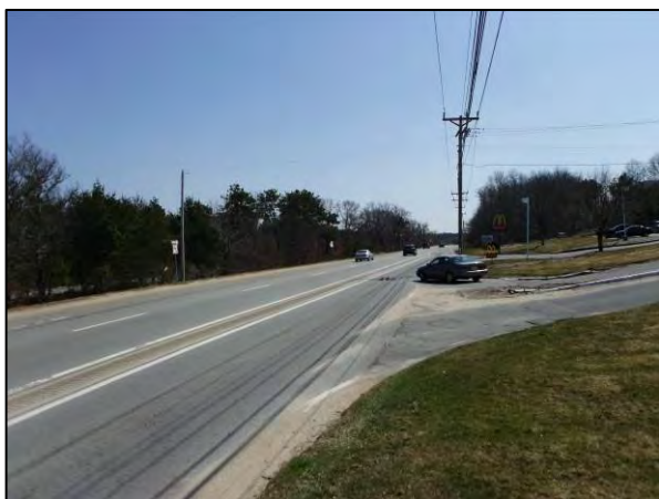
A flush concrete median separates Route 28 southbound through traffic and traffic entering and exiting commercial businesses in the vicinity of Clay Pond Road.
