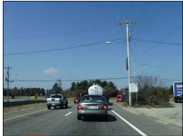
There is no advanced guide signage indicating the possible exits from the rotary.
