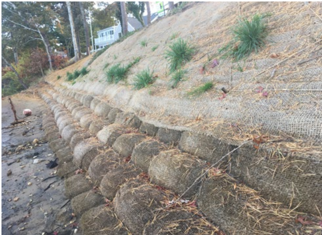
Fiber rolls help stabilize the toe of the slope that may be eroding due to wave action, until vegetation is established.
