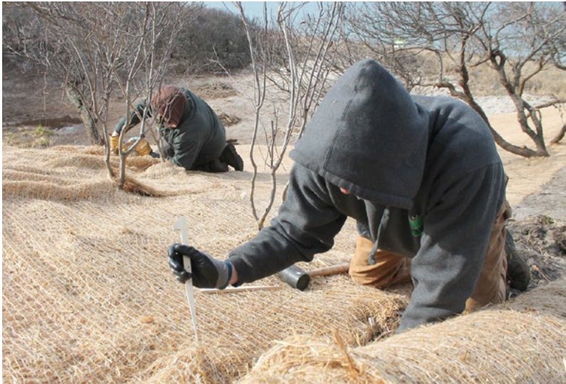
Blanketing slopes with biodegradable erosion control fabric holds soil in place while plant roots are establishing.
