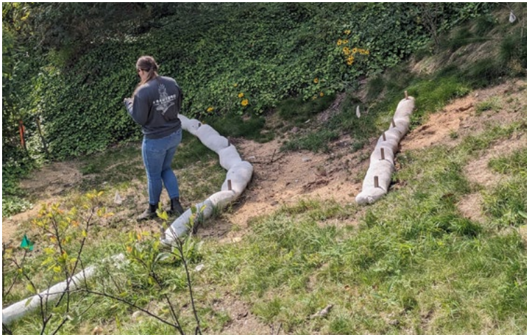
Filter socks help catch sediments in erosion-prone areas before they reach resource areas.
