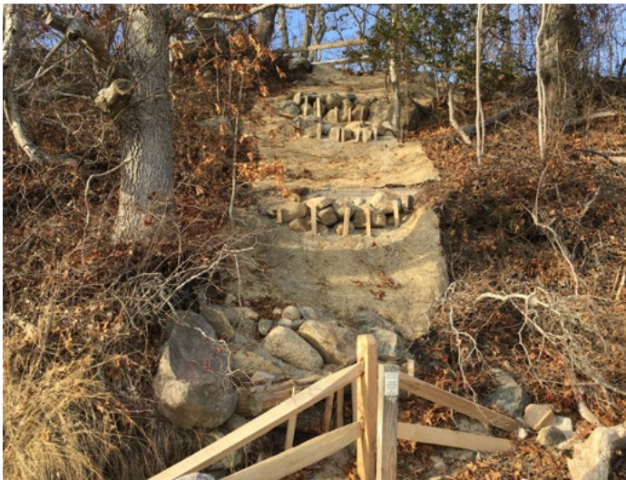
Check dams are a more permanent solution, but are also typically used in combination with plantings.
