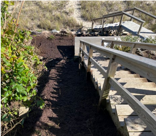
This narrow area along a set of raised steps is hydroseeded along with a flexible growth medium that temporarily stabilizes soil until the seed can germinate.
