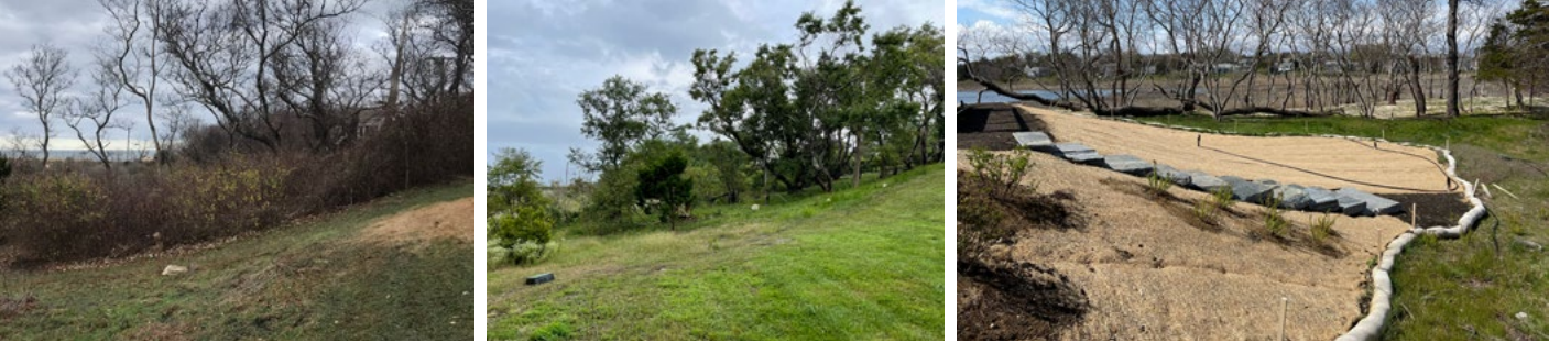
Year one: existing invasive plant material is removed, and the area is seeded. Areas that are disturbed from re-grading and new deck construction are blanketed and filter socks installed. Some of the shrubs have been planted through the erosion control fabric.
