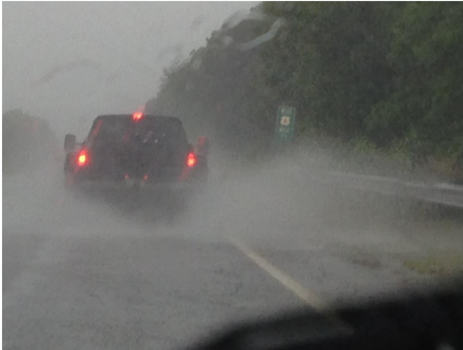
FIGURE 10: EAST OF EXIT 9 IN WESTBOUND LANE. PUDDLE COVERING ENTIRE DRIVING LANE.
