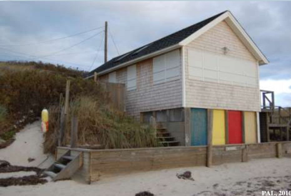
47 Pond Road, Cold Storage,, Truro
