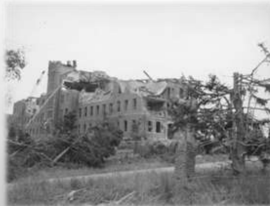
Tornado damage, 1953 Assumption College, Worcester Courtesy: Massachusetts Historical Society
