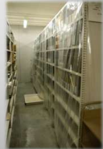
Roof leak Massachusetts Archives
