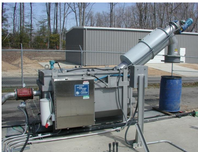
Figure 4-3 - Typical Package Septage Receiving Station (Courtesy of Lakeside Equipment Corp.)
