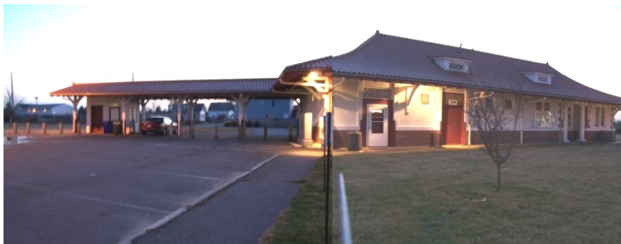
FIGURE 28. Former Rail Station in Buzzards Bay
