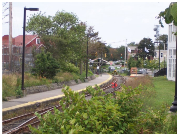
FIGURE 31. Rail Platform at the Hyannis Transportation Center
