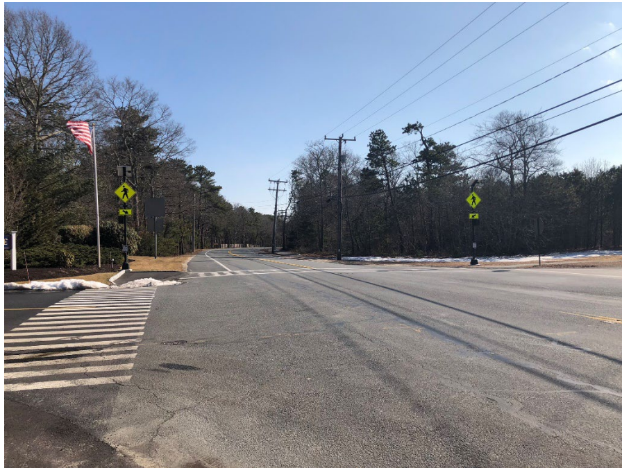
FIGURE 27. Rectangular Rapid Flashing Beacon located at the intersection of Great Neck Road South at Donna's Lane in Mashpee
