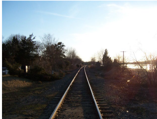
FIGURE 29. Rail Tracks West of the Sagamore Bridge
