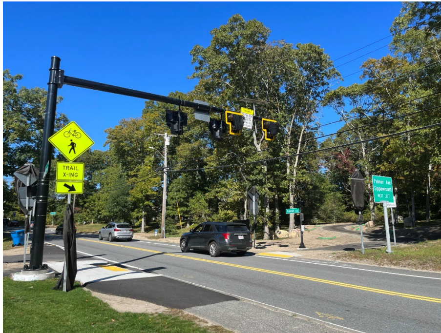
FIGURE 28. Pedestrian Hybrid Beacon located on Route 28 in Falmouth which provides a connection between the Shining Sea Bikeway and Goodwill Park
