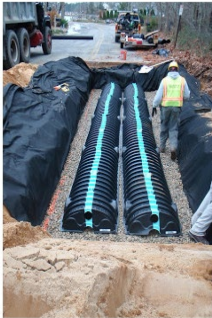
FIGURE 13. Sub-surface Treatment Chambers
