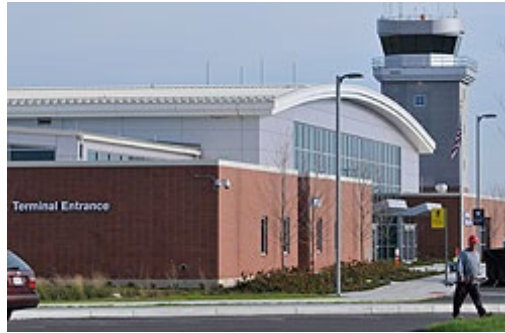
FIGURE 34. Barnstable Municipal Airport Terminal
