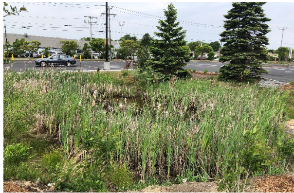
Figure 32. Bioswale/Rain-Garden in at the Hyannis Transportation Center
