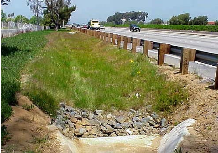
FIGURE 17. Water Quality Swales
