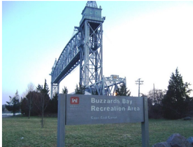
FIGURE 27. Cape Cod Canal Rail Bridge
