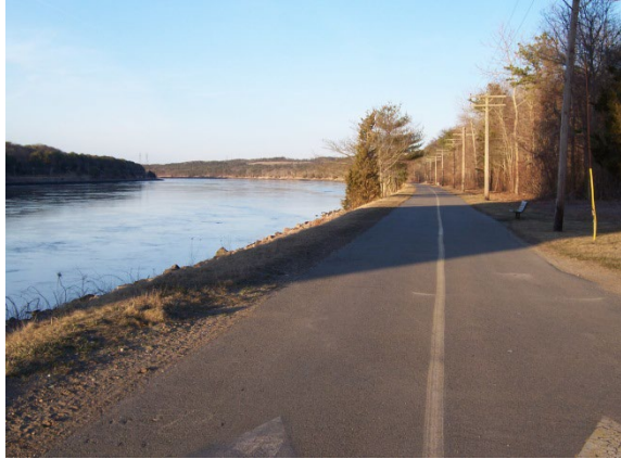
FIGURE 9. Southern-Side of the Canal Bicycle Path, East of Sagamore Bridge
