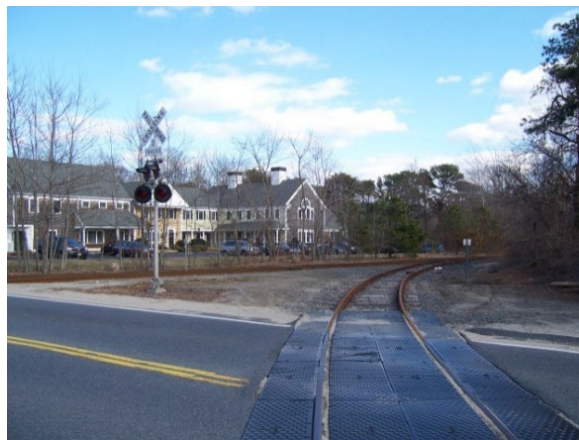
FIGURE 30. Rail Crossing at Willow Street in Yarmouth
