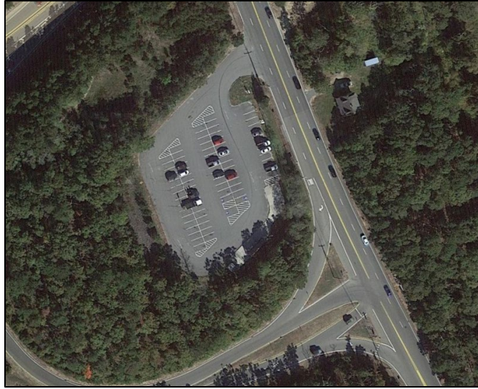
FIGURE 16. Harwich Park and Ride Lot On Route 124
