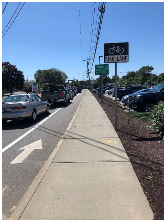
FIGURE 22. Bicycle lanes on Route 28 (North of the Jones Road Intersection) in Falmouth
