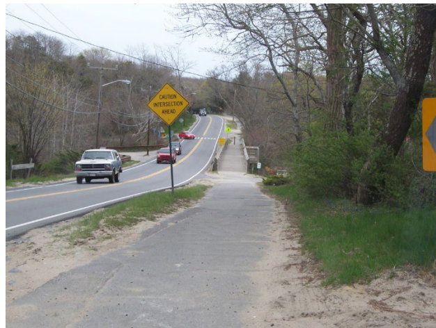
FIGURE 17. Looking South on Route 130 Bicycle Path at Lovell's Lane, Mashpee
