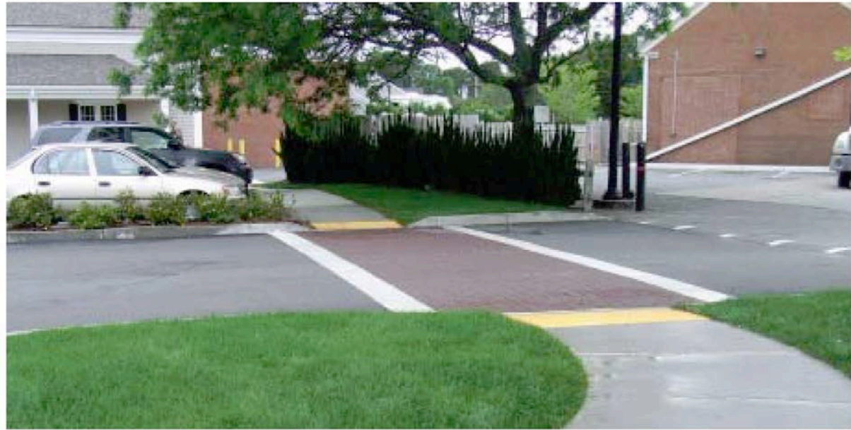
Detectable warning strip at pedestrian crossing at Crowell Road in Chatham.
