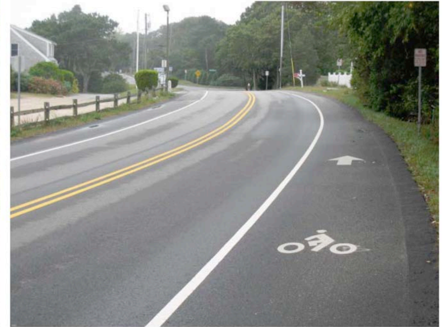
Bicycle lane with pavement markings on George Ryder Road in Chatham.
