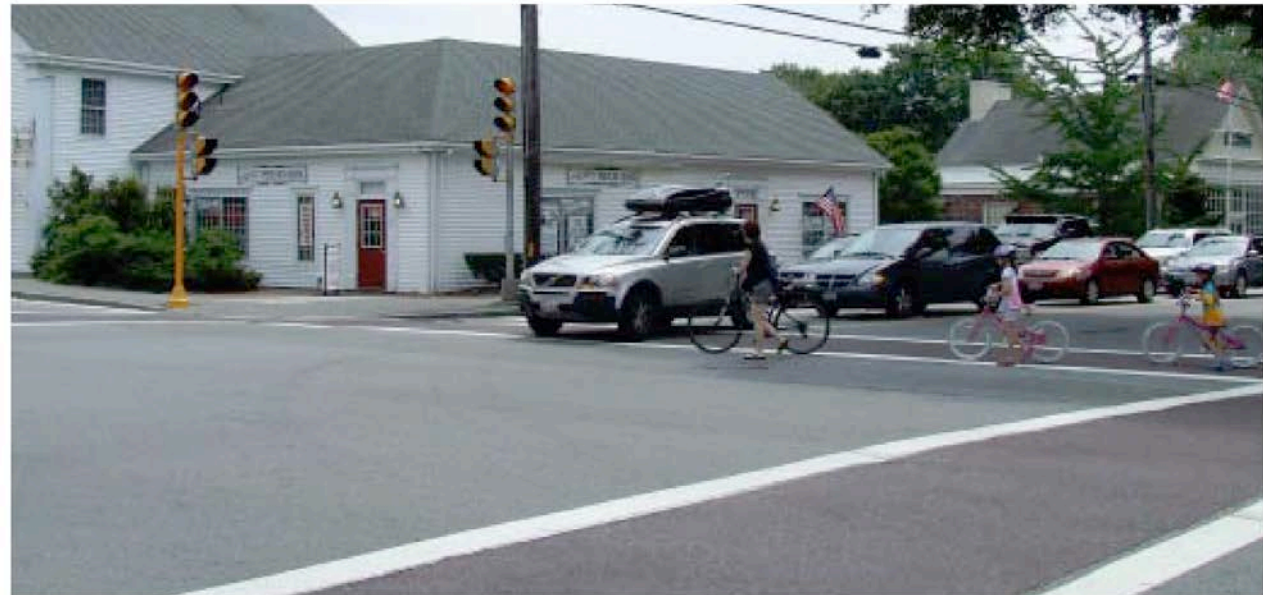
Tighter corner radii on Route 6A in Orleans shorten crossing distances.
