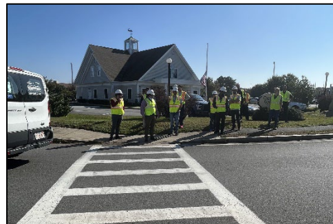
Image 9: No pedestrian equipment on the sidewalk in the southeast quadrant to allow pedestrians to start the pedestrian phase.
