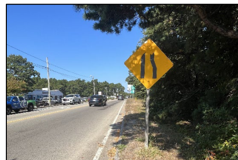
Image 6: Existing W4-2 lane drop signs that were inadvertently located on Station Avenue.
