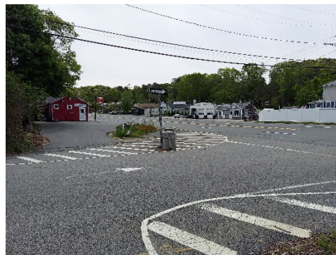
Image 7: Adams Street SB Single wide lane approach operates as two lanes
