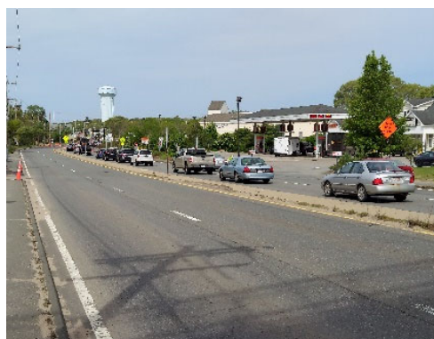
Image 1: Lack of shoulder or right turn lane by the Speedway Gas Station
