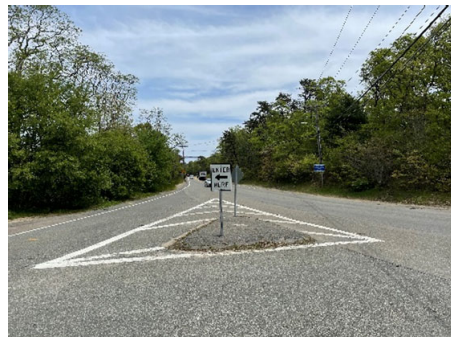
Image 3: Signs obstruct sightlines to east, from stopped approach
