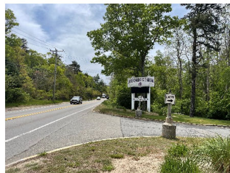
Image 5: Vegetation was observed obstructing sightlines to the entrance to Gallo Arena
