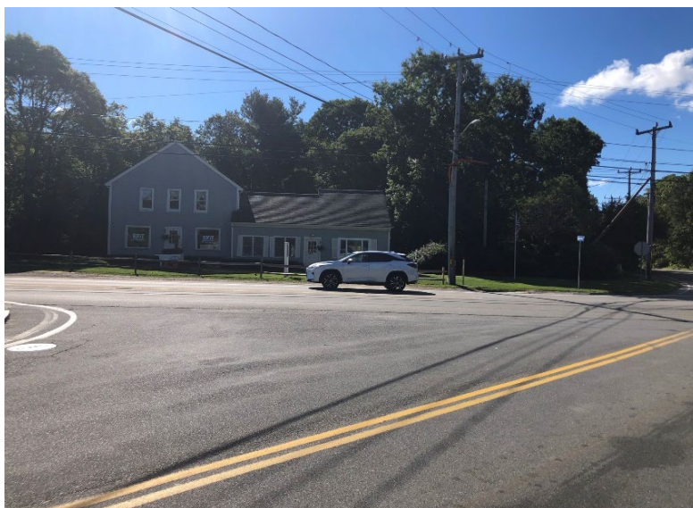
Image 3: A view of the wide corner radii in the northeast corner of the intersection
