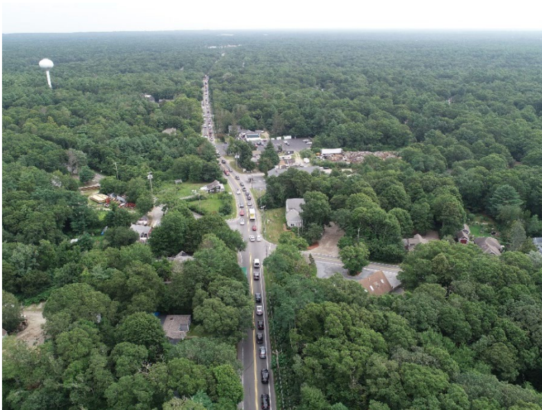
Image 1: Route 28 congestion (drone view looking east)
