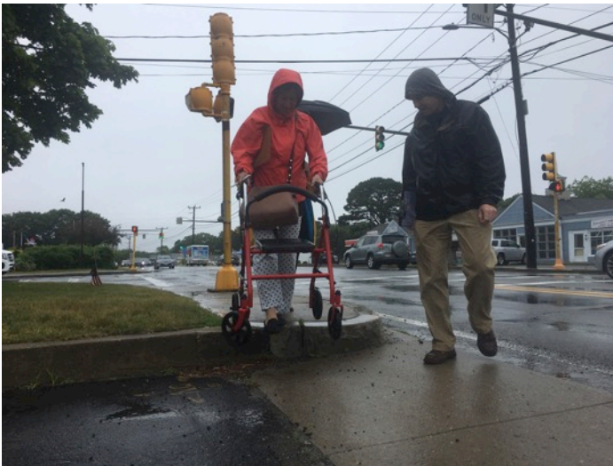
Example of a typical curb condition along Route 28.
