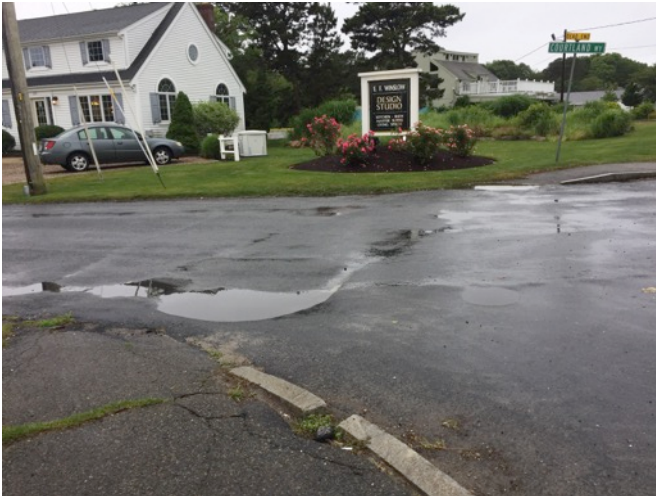
Crosswalks are not painted across town-owned streets that intersect Route 28.
