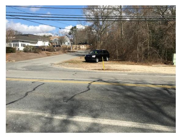
Figure 8– Car blocking sight distance on northeast corner of intersection
