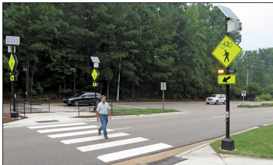
Figure 15- Crossing equipped with Rapid Flash Beacons
