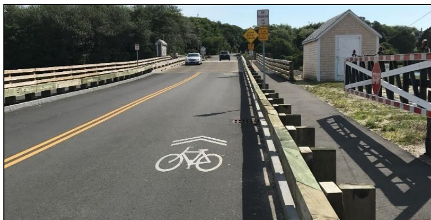
Figure 13 - "Sharrow" Pavement Marking on Bridge Street in Chatham
