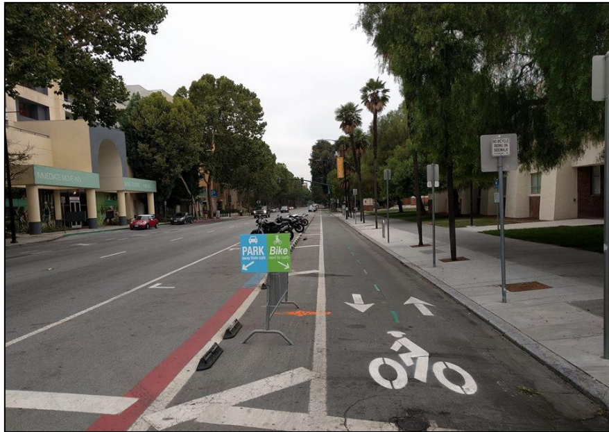
Figure 14 - Conversion of Motor Vehicle Lane to Bicycle Path in San Jose
