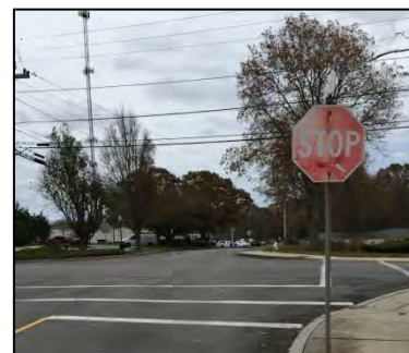
Image 8: Faded stop-sign along the Spring Bars Road eastbound approach.
