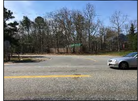
Image 13: Missing stop bar on Northbound Sam Turner Road approach
