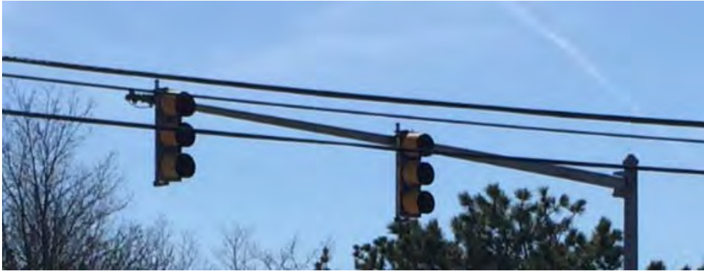
Figure 10 - Potential obstructed view of signal housings due to utility cables
