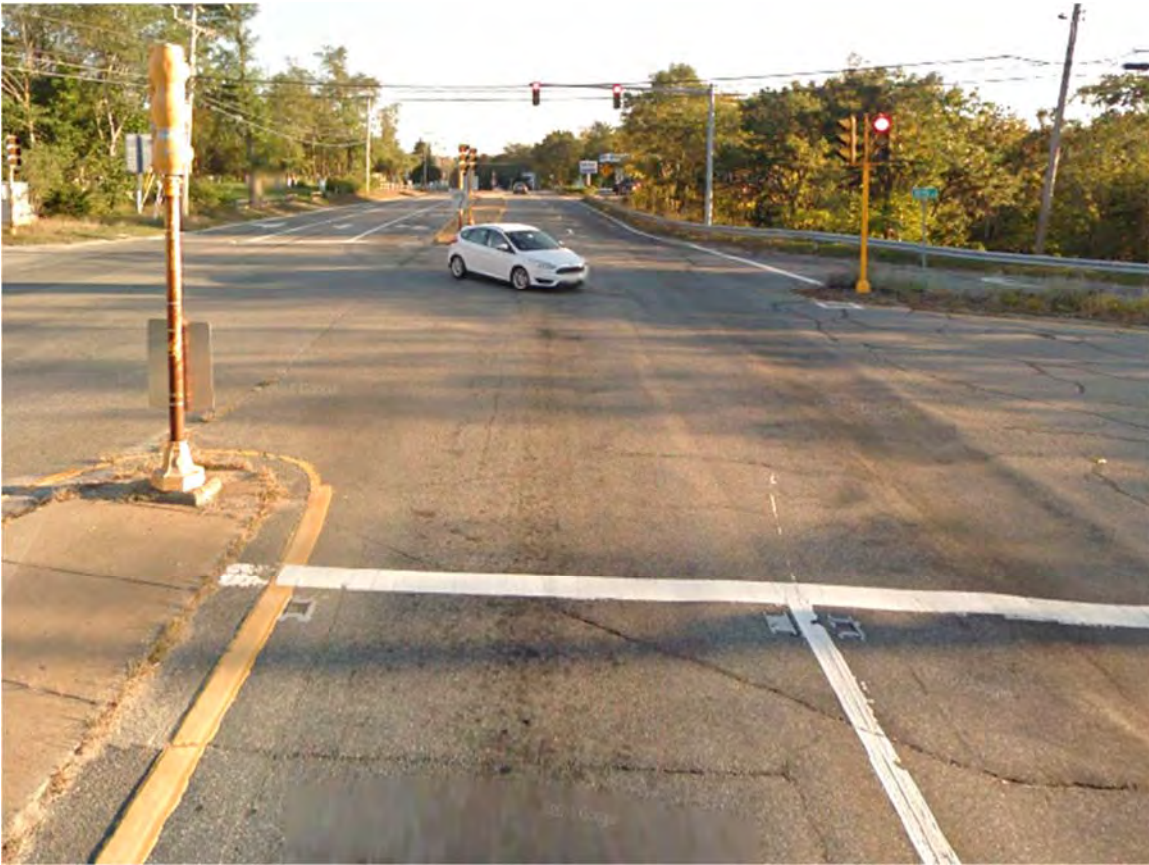
Figure 9 - Looking south -note oncoming left turn lane (when occupied) obscures view of southbound left-turning motorists
