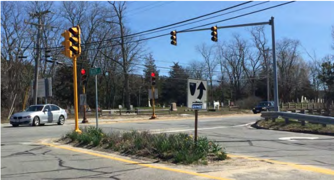
Figure 8 - Looking east from Main Street - note low height of "Keep Right" signs
