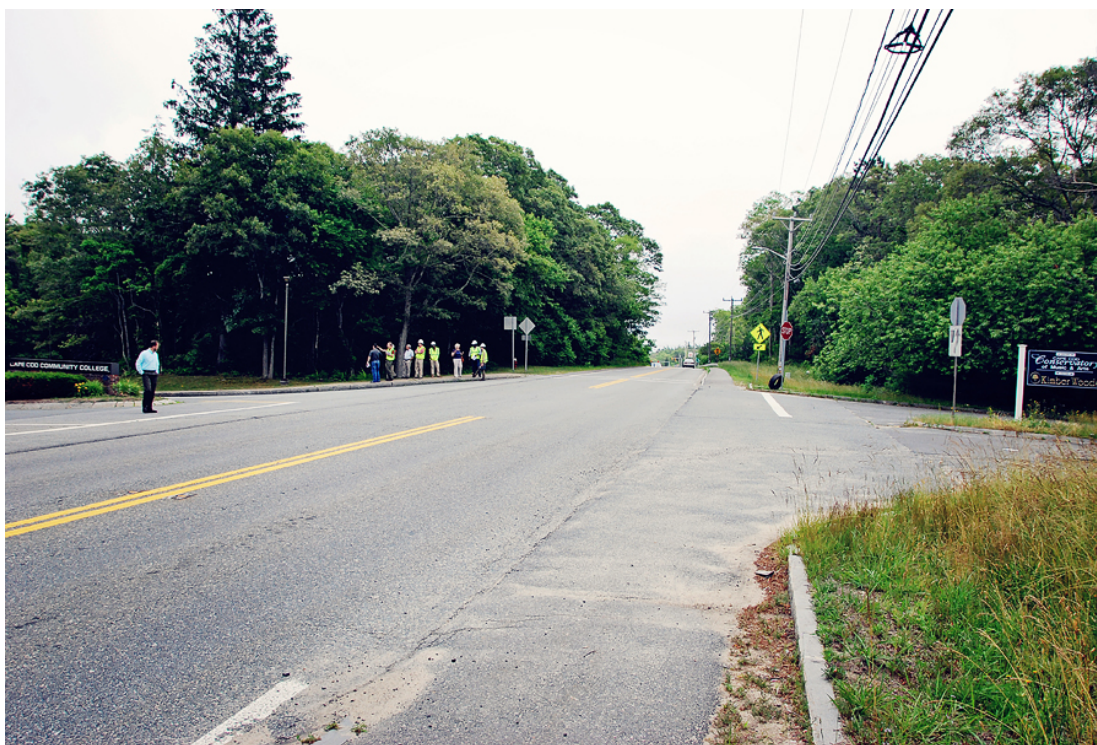
Figure 4 - View of Route 132 traveling southbound
