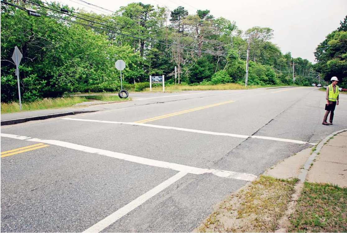
Figure 9 - View of crosswalk markings across Route 132
