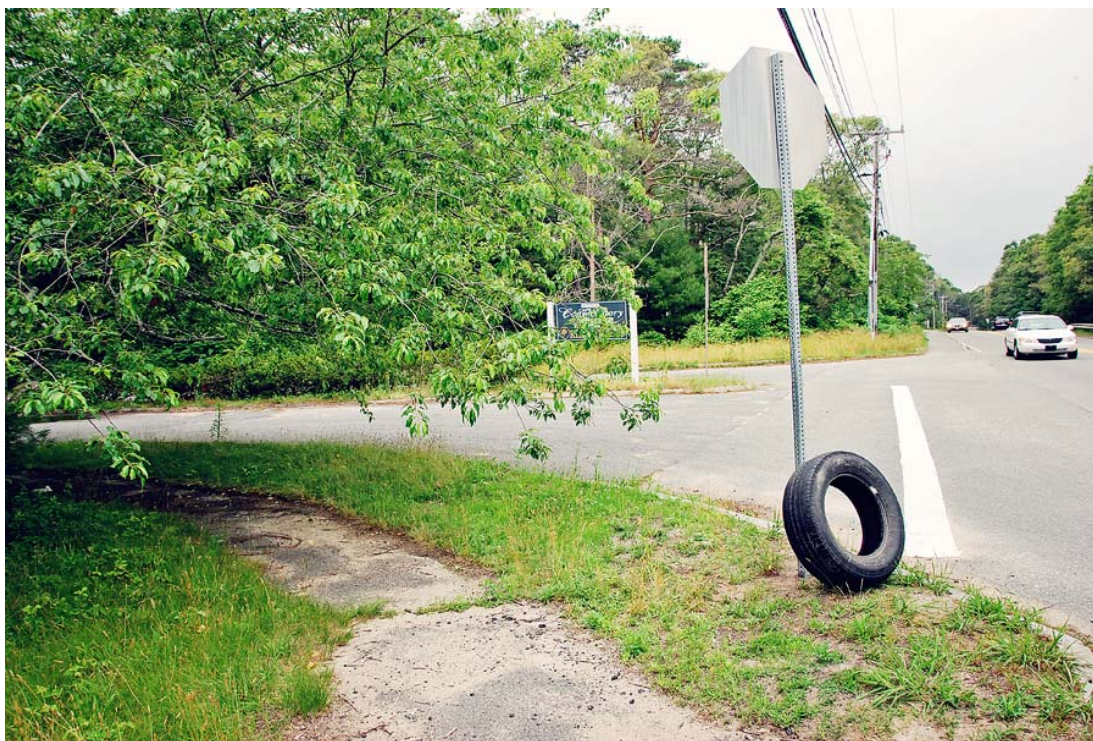
Figure 8 - View of sidewalk turning into the Cape Cod Conservatory of Music & Art. This view also depicts the evidence of no crosswalk and no accessible ramps for pedestrians
