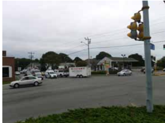
No overhead signal indications facing the Yarmouth Road northbound approach.
