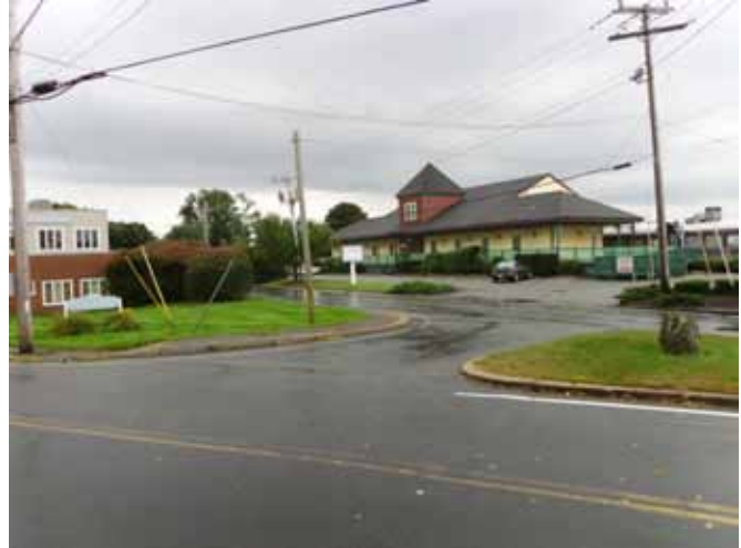
Slip lane between Yarmouth Road and Camp Street
