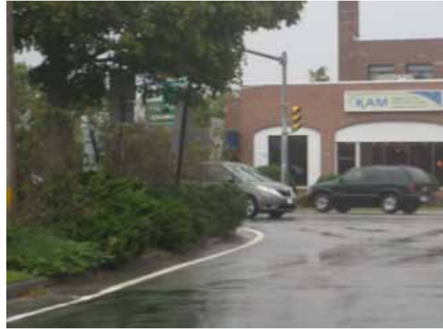
Guide signs facing Yarmouth Road the northbound approach are blocked by trees.
