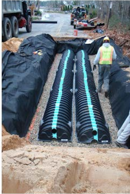
FIGURE 7. Sub-surface Treatment Chambers
