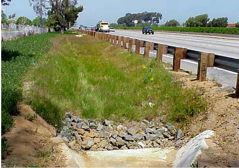
FIGURE 11. Water Quality Swales
