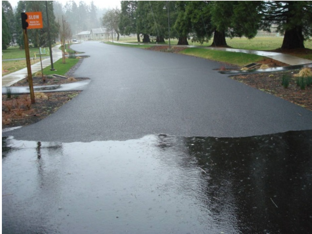
FIGURE 5. Porous Pavement adjacent to traditional impervious asphalt pavement (foreground)
