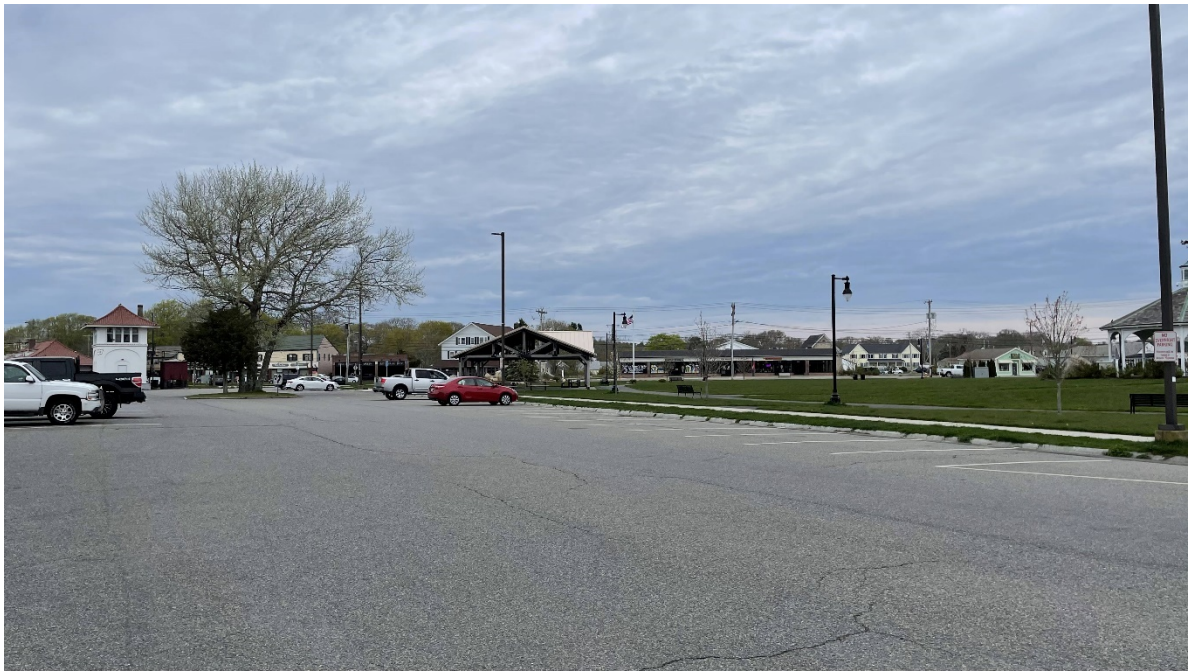
Parking area next to Buzzards Bay station building
