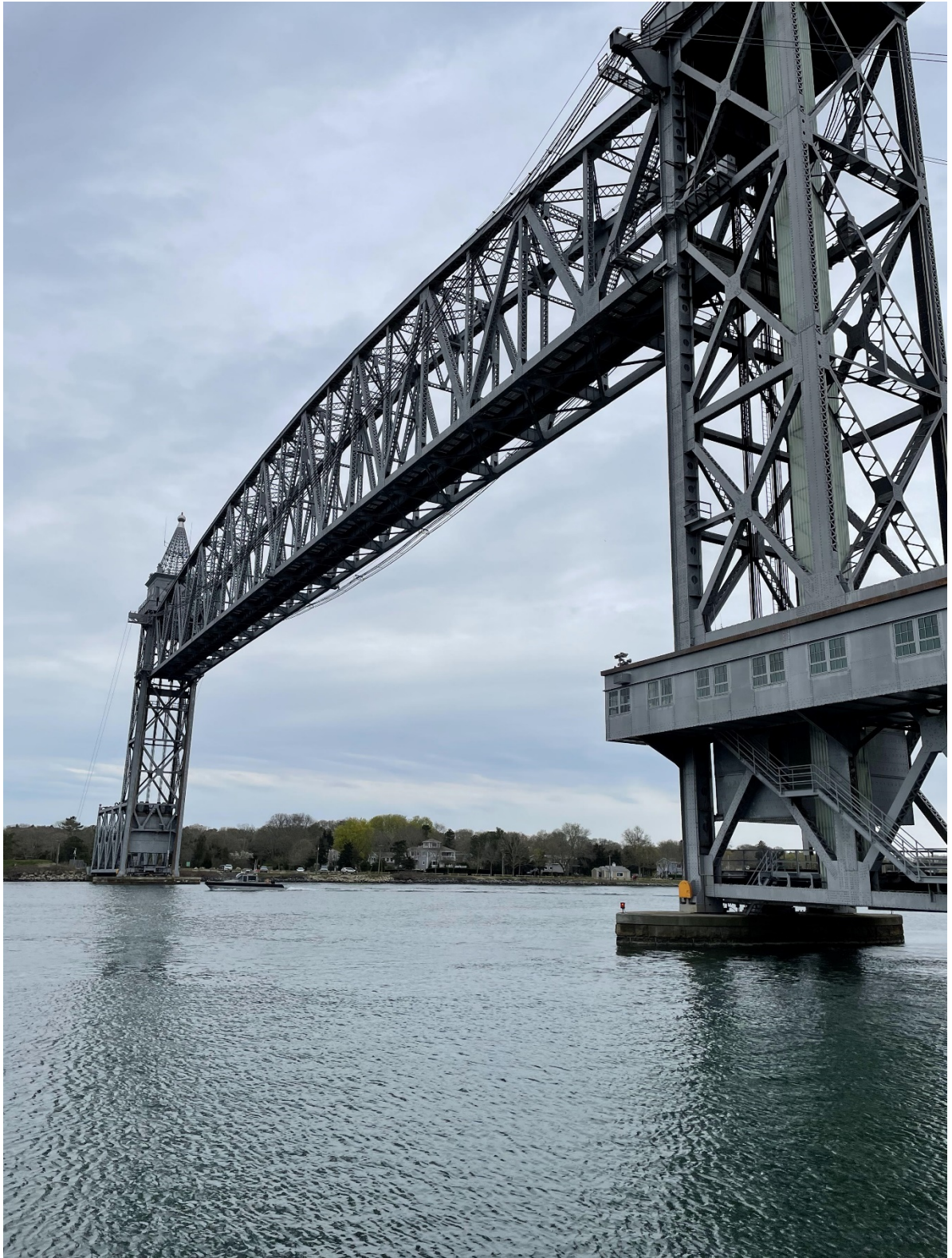
Cape Cod Canal Railroad Bridge
