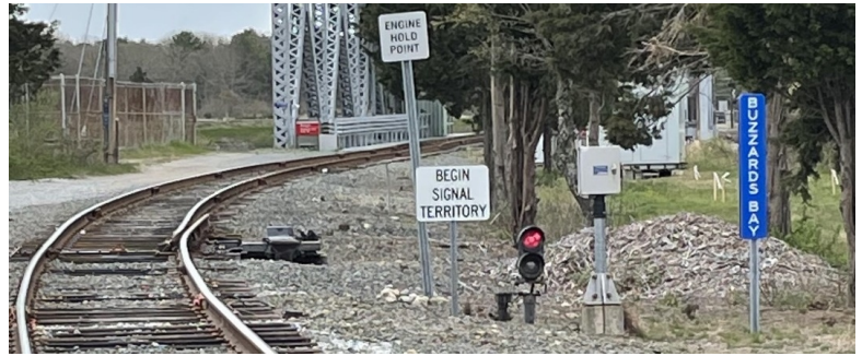
Signals near the Cape Cod Canal Railroad Bridge
