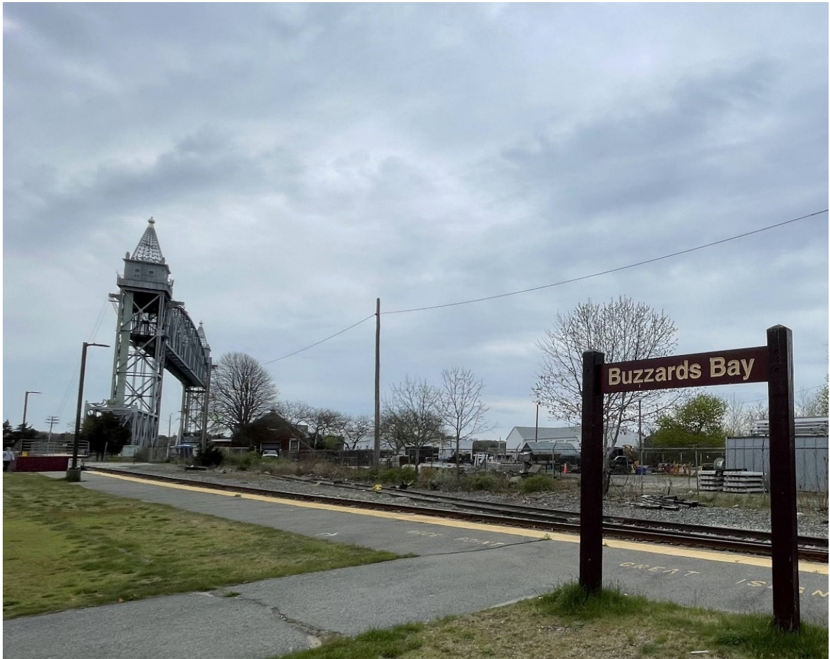
Existing station at Buzzards Bay
