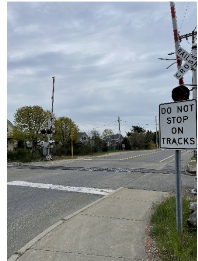
Grade Crossing at Academy Drive just north of Buzzards Bay station
