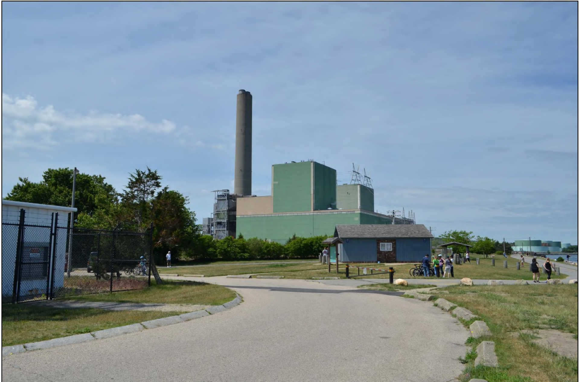
Figure 5.A-9a Entrance to USACE Public Walkway – Before
