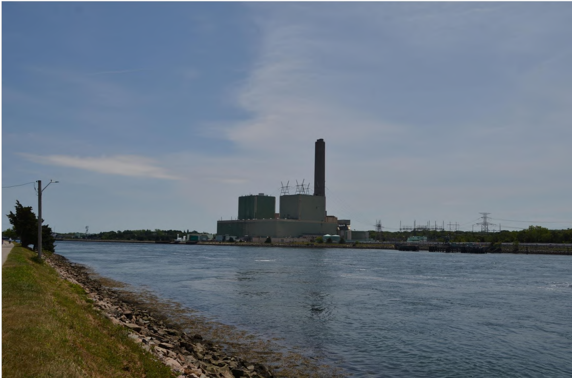
Figure 5.A-17b Scusset Beach Road Pier – After
