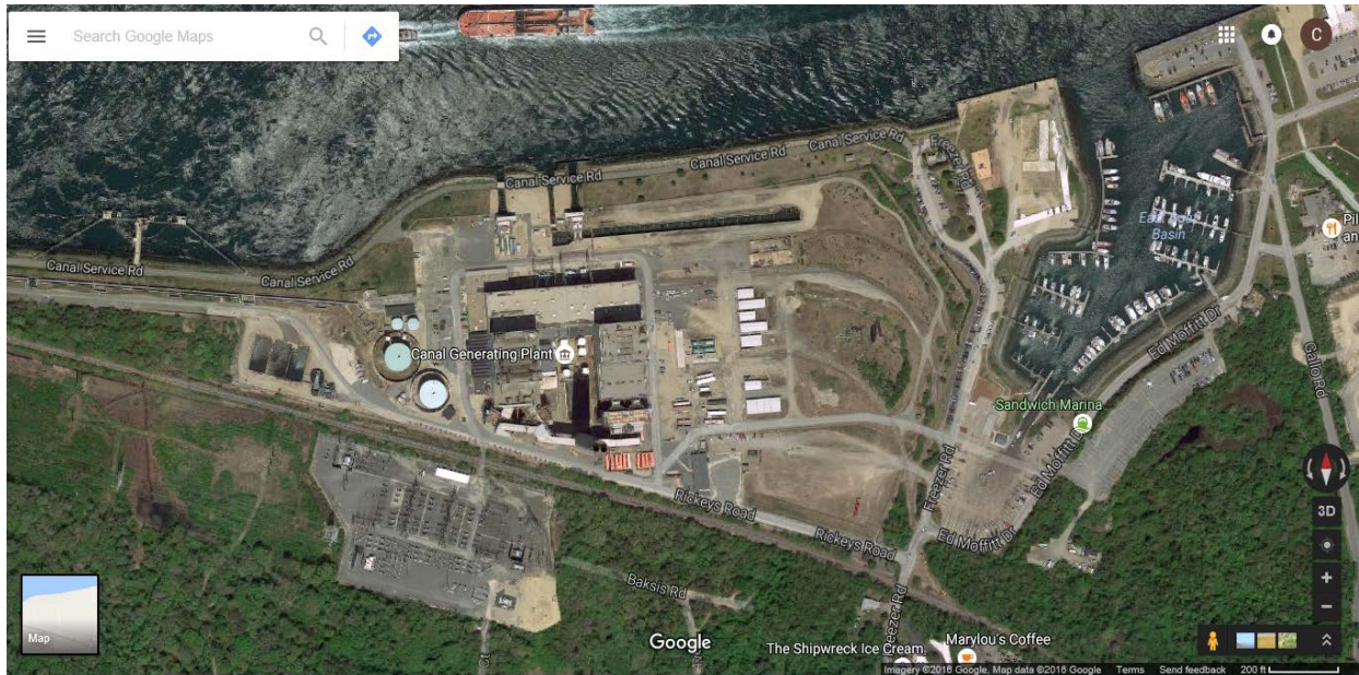
Figure 1 Aerial View of Existing Canal Generating Station, Sandwich, Massachusetts
