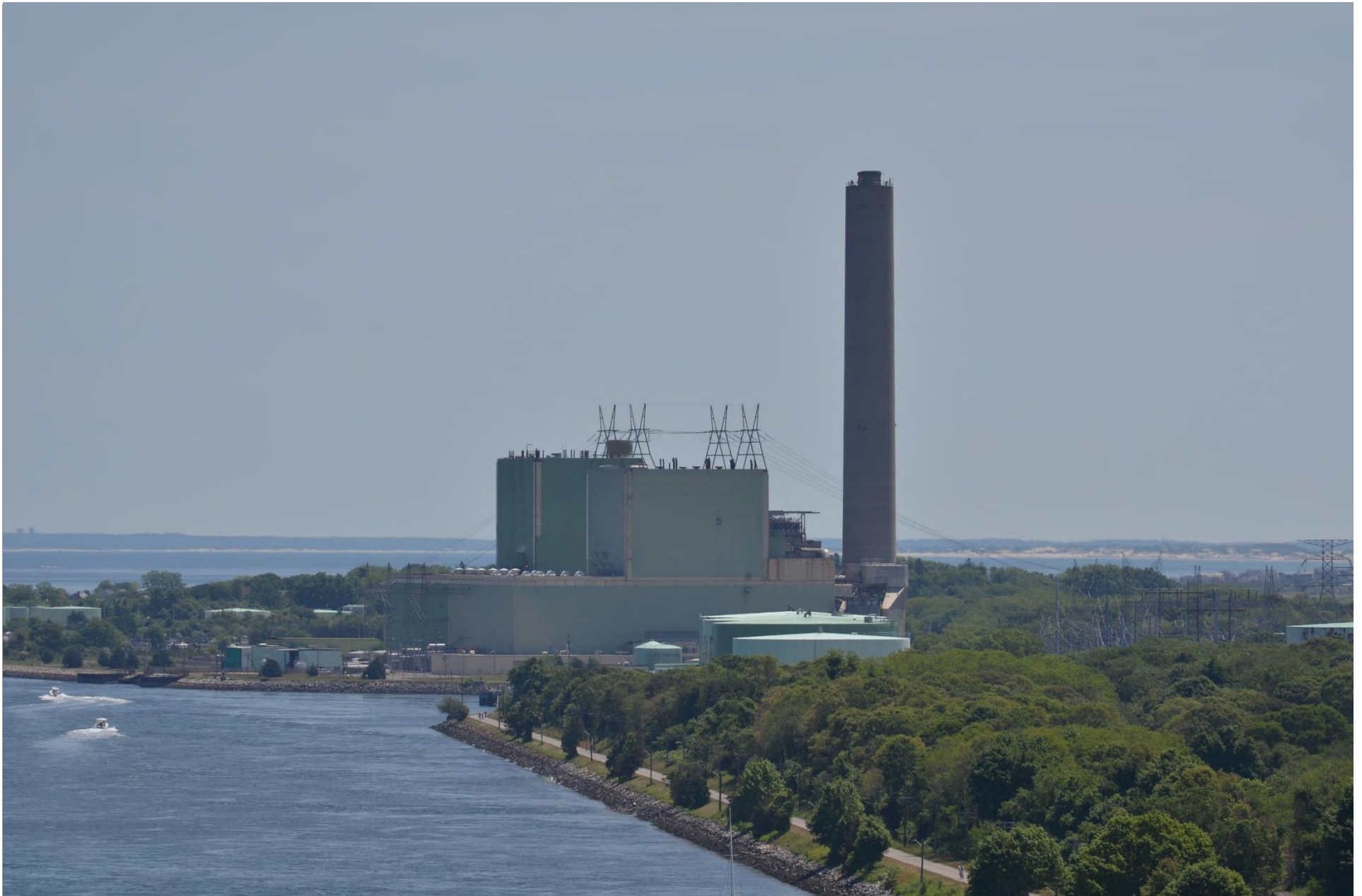
Figure 5.A-15b Sagamore Bridge – After
