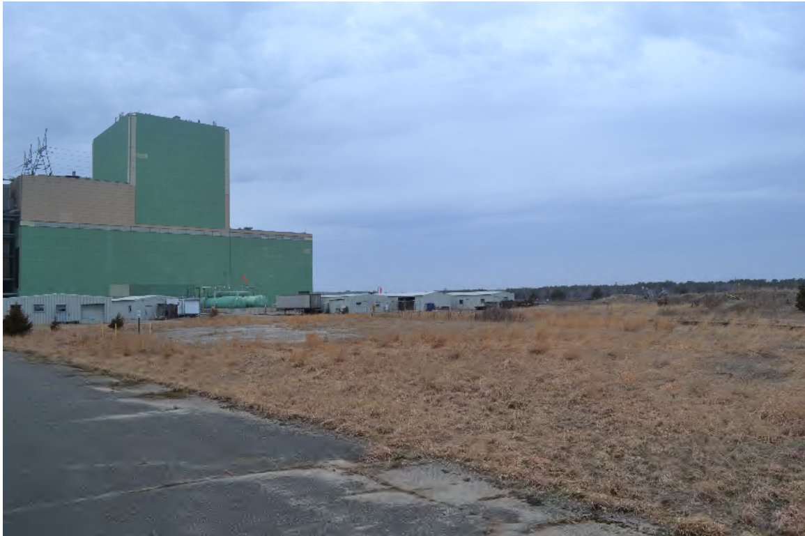
Photograph 2. The Project Site (view toward the northwest)
