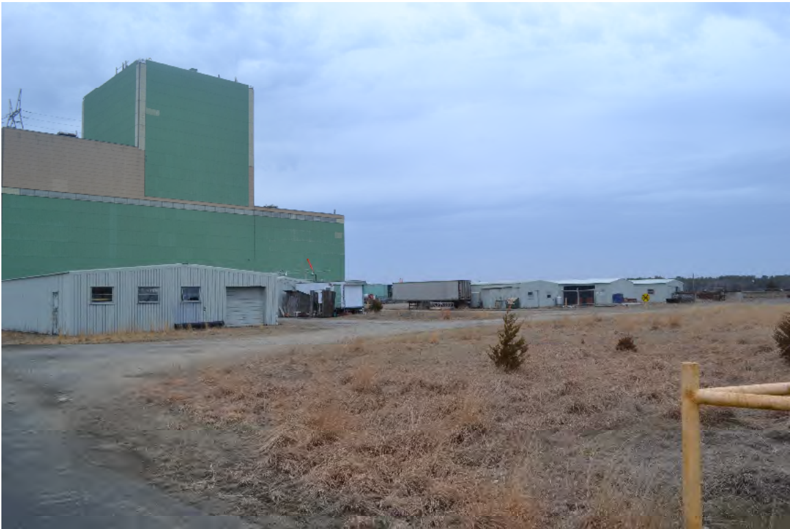
Photograph 3. Warehouses to be demolished (view toward the northwest)
