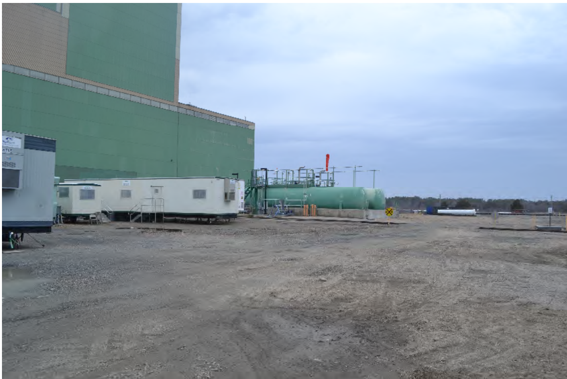
Photograph 4. Ammonia tanks & trailers to be relocated (view toward the northwest)
