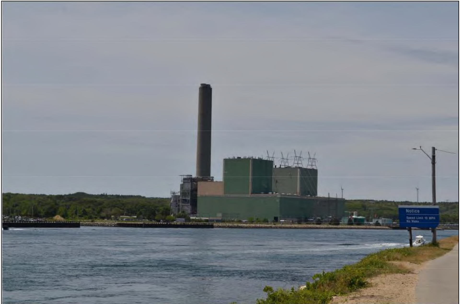
Figure 5.A-16a Scusset Beach Parking – Before
