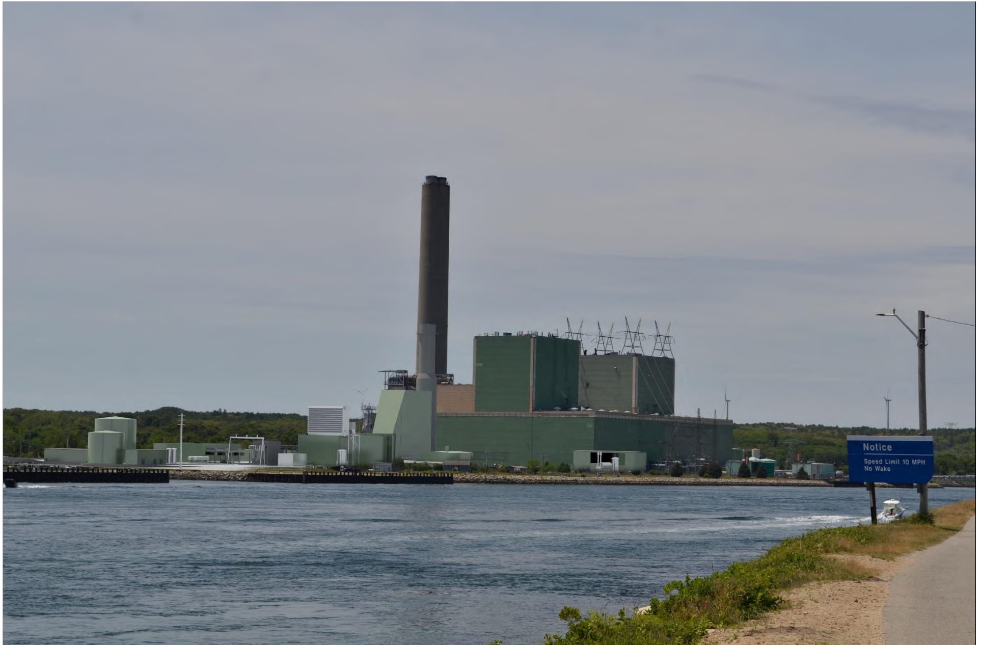
Figure 5.A-16b Scusset Beach Parking – After
