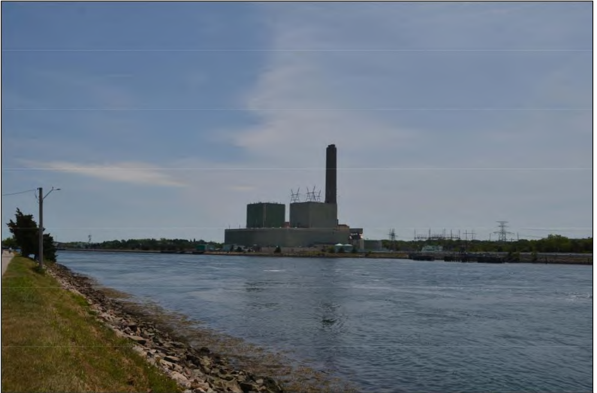
Figure 5.A-17a Scusset Beach Road Pier – Before
