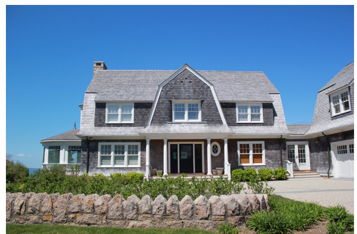
Example of modern construction on Chapoquoit Island which incorporates elements of Shingle style such as a cross gambrel roof and wood shingles
