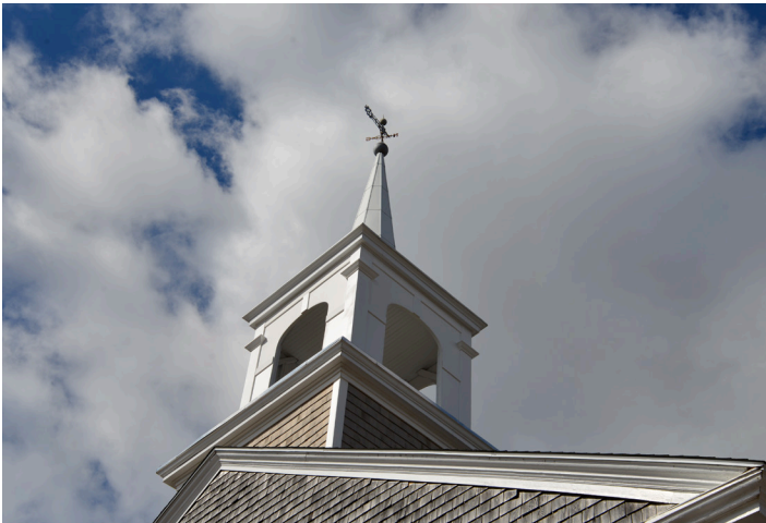
The East End Meeting House's steeple, which was added in the 1840s, was replaced with a fiberglass replica in the 1980s to alleviate pressure on the roof.
