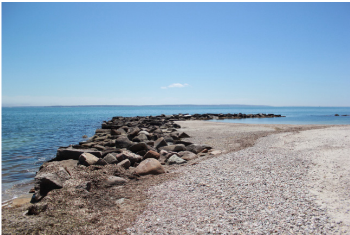
Detail of Old Stone Wharf
