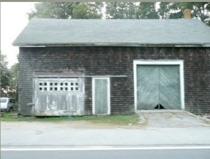
Siting and condition
