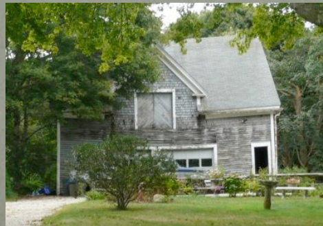
Siting and condition
