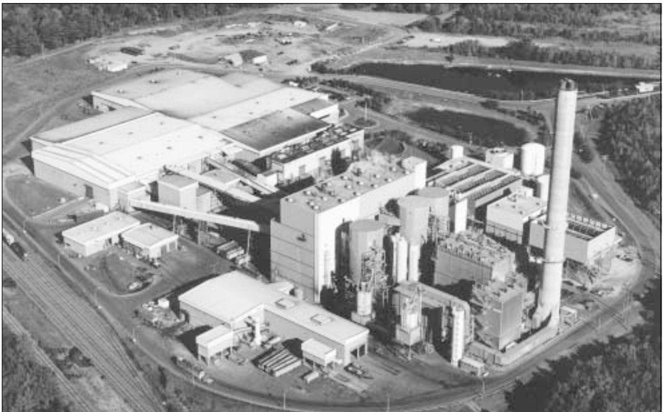
The SEMASS waste-to-energy facility in Rochester, Massachusetts.
