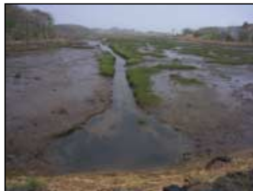
The seaward marsh area is degraded, displaying vegetation die off, ponded water, and a major scouring basin.
