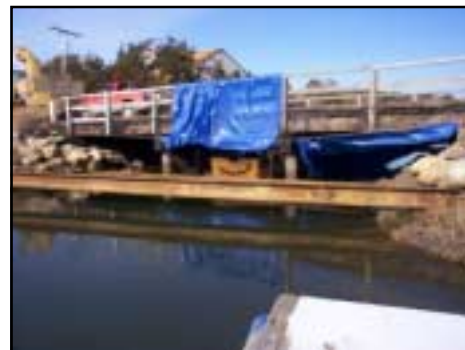
Construction underway on the Santuit River bridge to widen and raise the roadway; unfortunately plans do not include alleviating the restriction.
