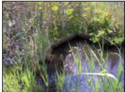
This concrete headwall houses the upstream opening of the 30 inch pipe passing under Route 6. Stagnant water obscures the submerged pipe.
