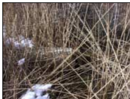
Corrugated metal pipe with flapper gate visible through the Phragmites at the seaward opening of BR-3.
